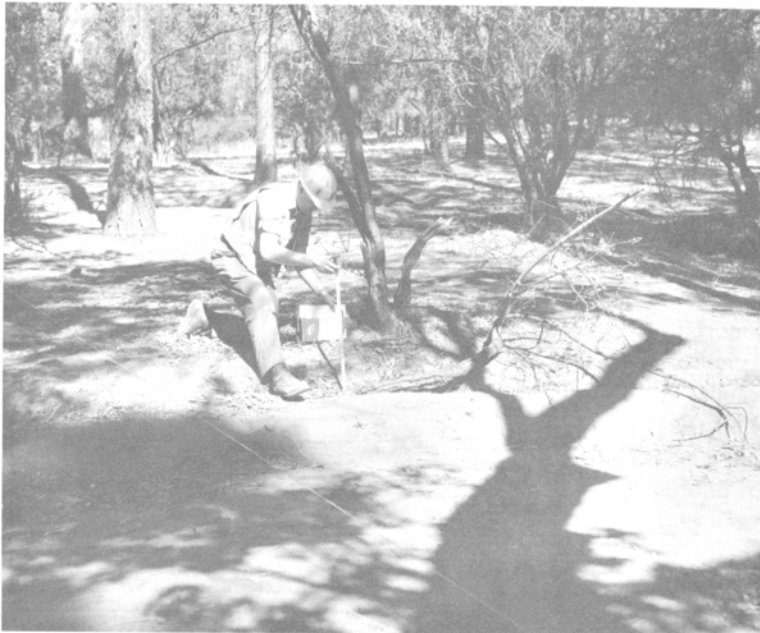
Figure 10—Bare areas occur where campers have prepared tent foundations. Sharp cuts and fills slough away as the site is used.
