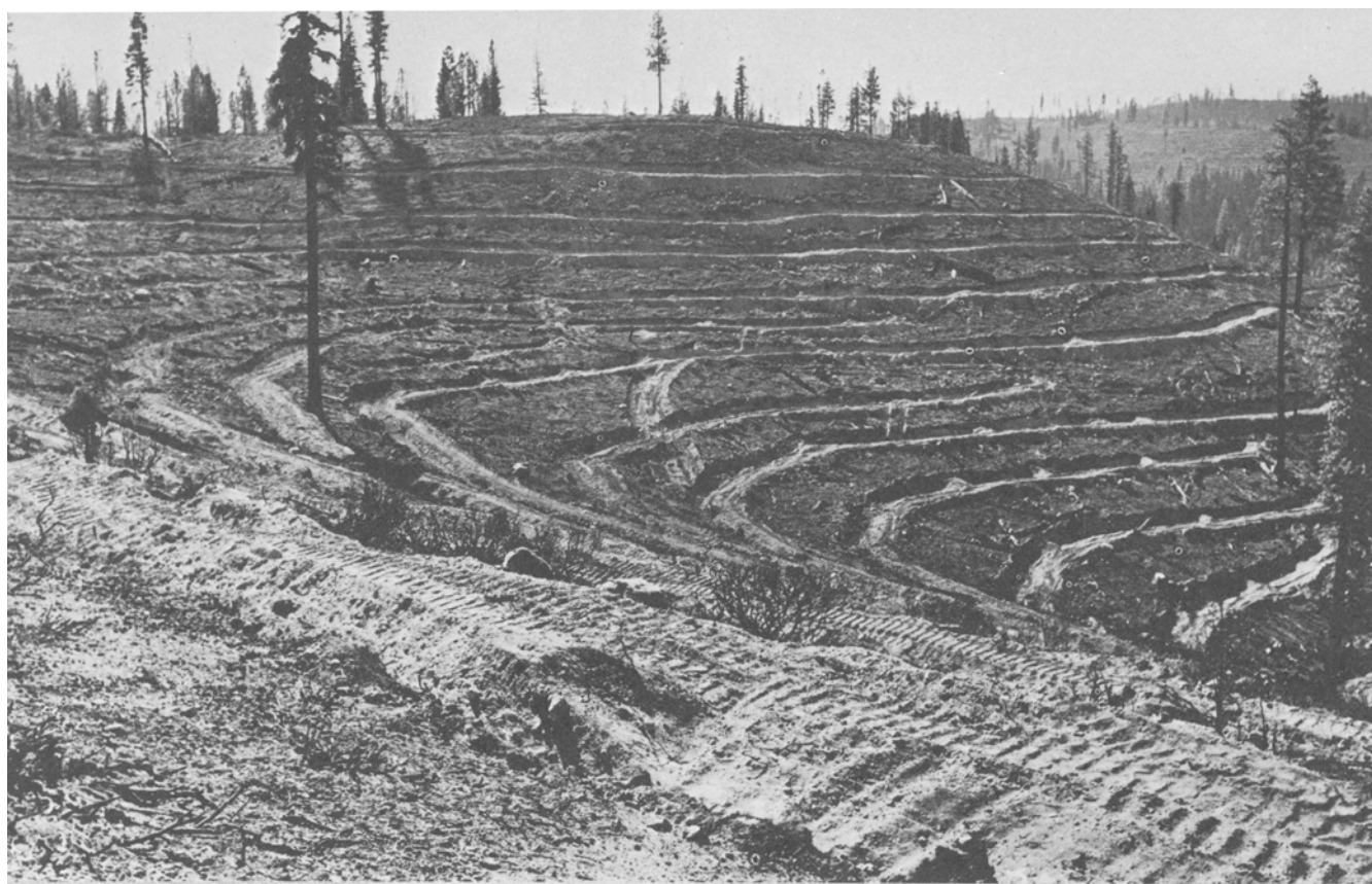
Figure 12.—Contour trenches at the Tahoe National Forest are being tested in research on runoff and erosion prevention. Studies are being made on the effects of forest fires and the effectiveness of four alternative treatments on flood peaks, sedimentation, snow storage, and soil moisture loss.
