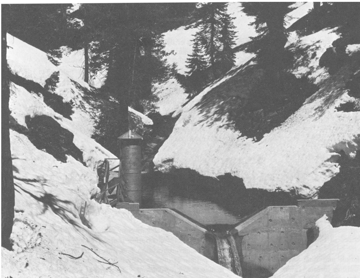
Figure 13.—Water yield resulting from application of alternative management techniques will be tested on a dozen small watersheds with weirs.
