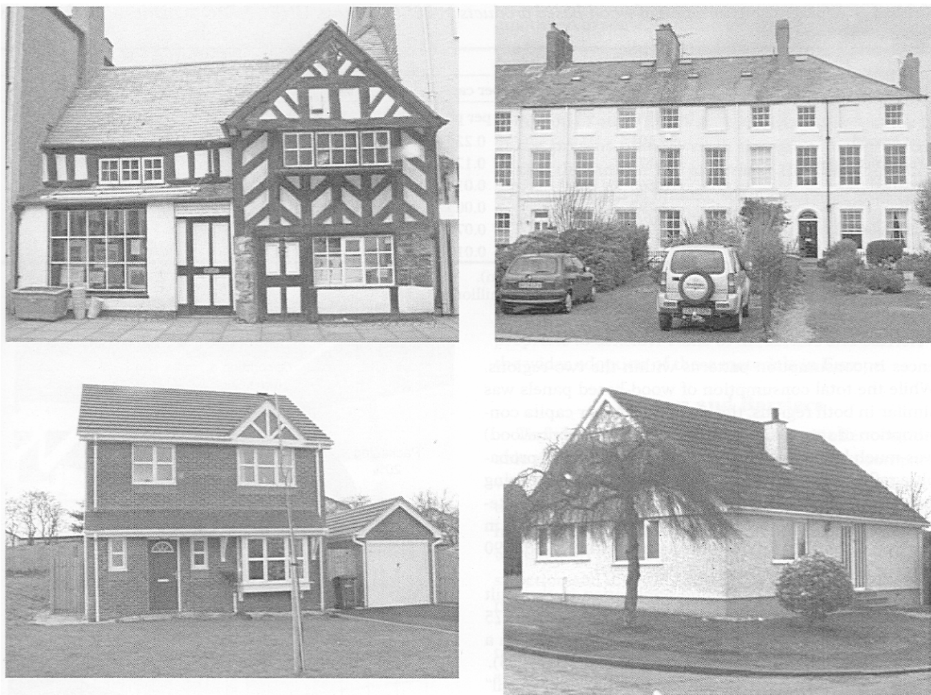
Figure 3. – Some examples of residential construction in the United Kingdom from circa 15th–17th century (top left), 18th century (top right), and late 20th century with either a brick (bottom left) or render (i.e., cementitious stucco) over masonry block construction
