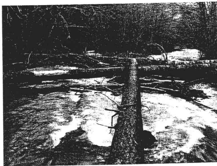
FIGURE 13.5. Large wood restoration in a coastal Oregon stream. Log jams were placed where they could increase the stream's connections with its floodplain during moderate stream flow. (Photo by Jack Sleeper, Siuslaw National Forest)
