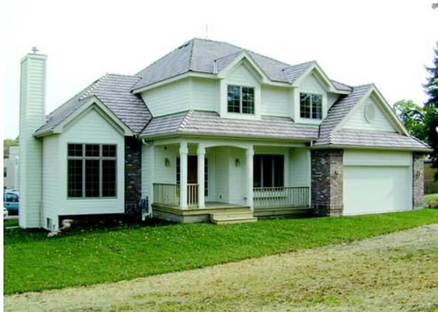
Figure 1 The FPL research house in Madison, Wisconsin.
