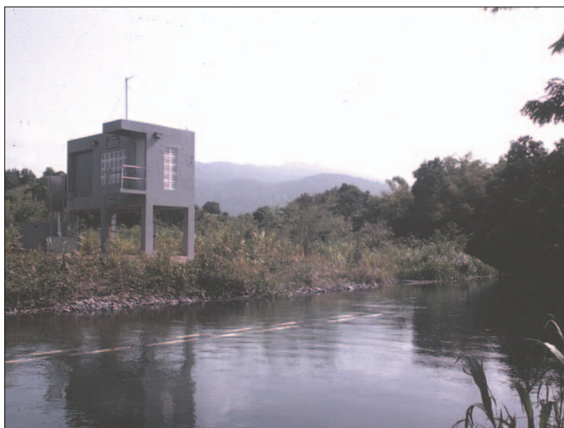
Figure 5. The in-channel withdrawal structure located on the Río Mameyes, Puerto Rico. Water is pumped from the submerged stainless steel risers to the pumphouse on the bank. Photograph: James March.
