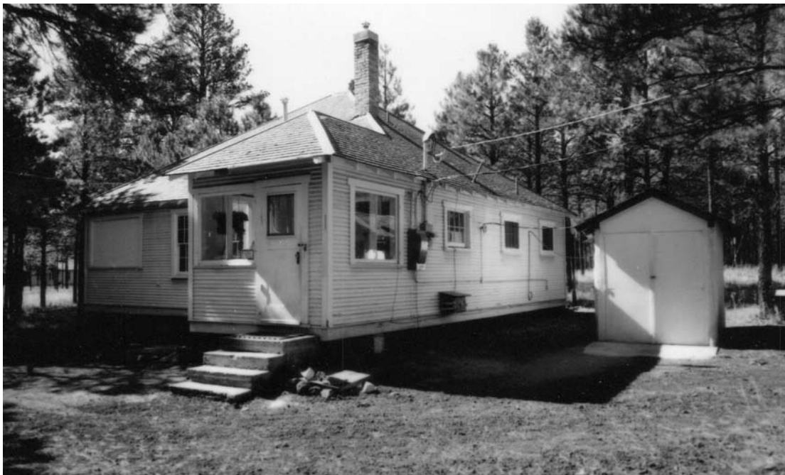
Figure 1. Main laboratory building at FVEF.
