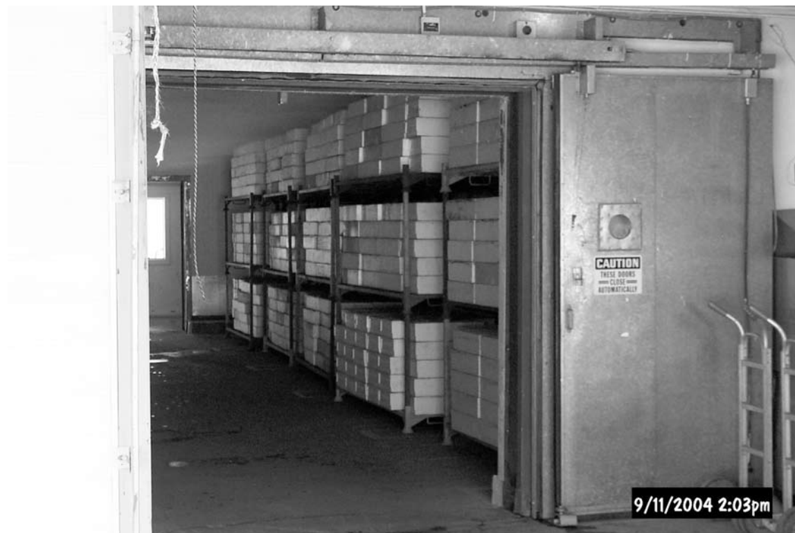
Figure 9 —A storage cooler was converted into a sterilization room. Steam pumped into the room provides high-humidity heat.
