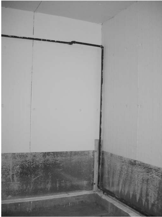
Figure 11 —Black pipe distributes steam in the sterilization room. The pipe runs along the bottom of the side walls. Steam leaves the pipe through holes (0.06 in [0.15 cm] in diameter) drilled into the pipe.
