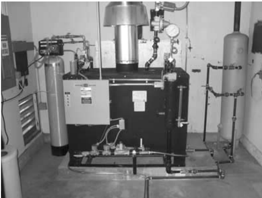
Figure 1 —This propane boiler supplies 160 °F (71 °C) steam to a 24 by 47 by 10 ft (7.3 by 14.3 by 3 m) room used to sterilize used Styrofoam™ containers.
