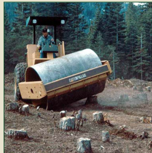
Compacting on a normal soil using a vibrating roller.
