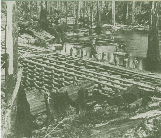
Splash dam storing water for a log run. For scale, note the men silhouetted by the water
