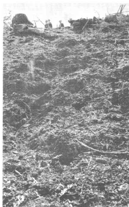
Figure 6.—Section of line in the light-medium slash with smaller fuels, left. The duff layer was 4 to 6 inches deep. Blasting, with 120 pounds of explosive, right, produced a 10-foot-wide break with a 2-foot mineral soil "trench" in the center.
