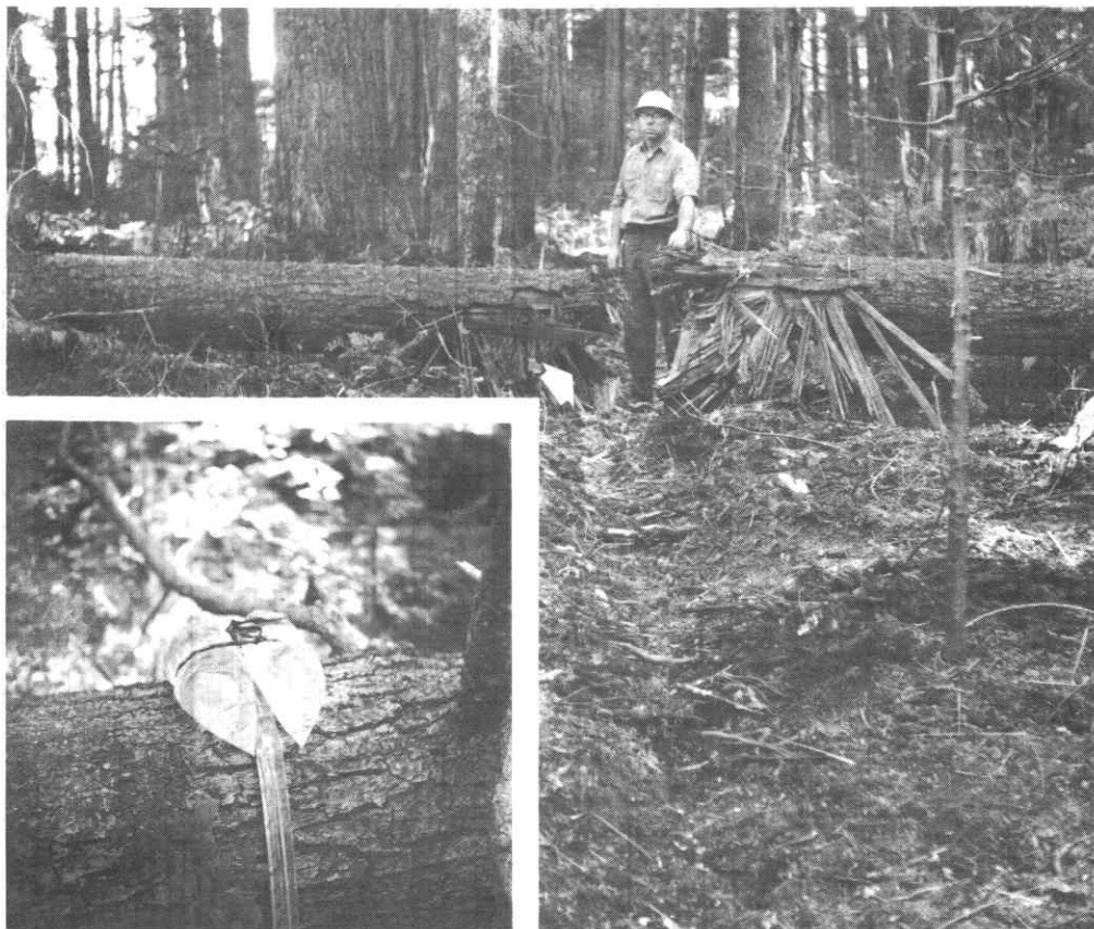
Figure 4.—An 18-inch log was blasted through by placing two 3-pound "satchel" charges in contact with the explosive-filled tubing where it crossed the obstruction.
