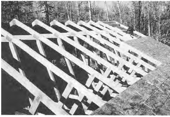
Figure 6.7. — OSB sheathing covering hard maple web demonstration trusses.
