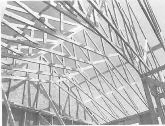
Figure 6.6. — Metal plate trusses containing red maple web lumber.
