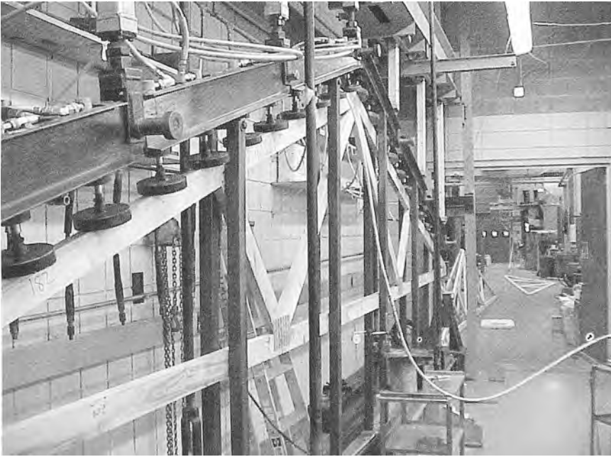
Figure 6.3. — Hardwood pitched chord truss during full-scale testing.
