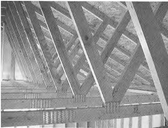
Figure 6.8.— Close-up of hard maple web, SPF bottom chord, and Douglas-fir top chord truss demonstration project.
