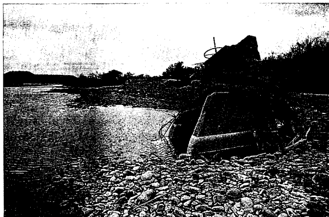
Figure 3.—High stagnation pressures from shooting flows of the unusual January 1979 flood in the Verde River, central Arizona, created uplift forces that aided in upsetting this water-diversion structure and a 2-foot-diameter concrete pipeline.
