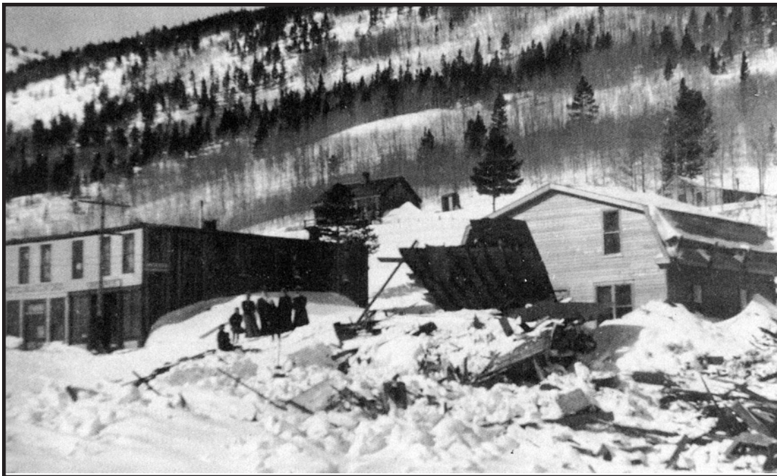
Figure 35. — Avalanche damage caused by the February 4, 1907, avalanche at Monarch. The flat-roofed building is the Blatchford Hotel mentioned in account 172A (John Ophus Collection, Salida).
