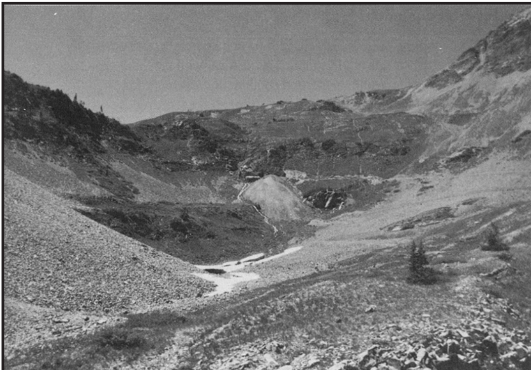
Figure 33. — The Augusta Mine from the near edge of the bench mentioned in Figure 32. Although the floor of the bench is relatively flat, the slopes above the road leading to the mine are steep and dangerous. This photo was taken in August 1981.
