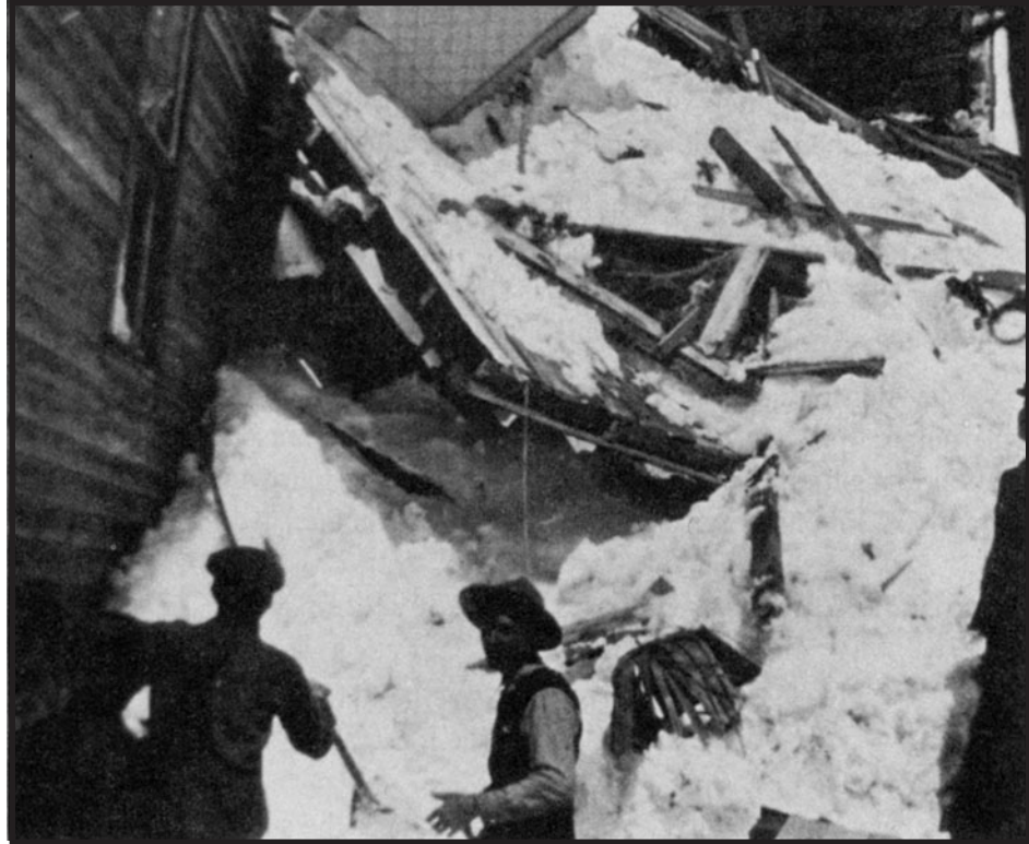
Figure 11. — Avalanche debris piled against the corner of the Town Hall at Silver Plume. This avalanche, which ran on April 23, 1921, flowed around the back of the Town Hall (Silver Plume Historic Society).
