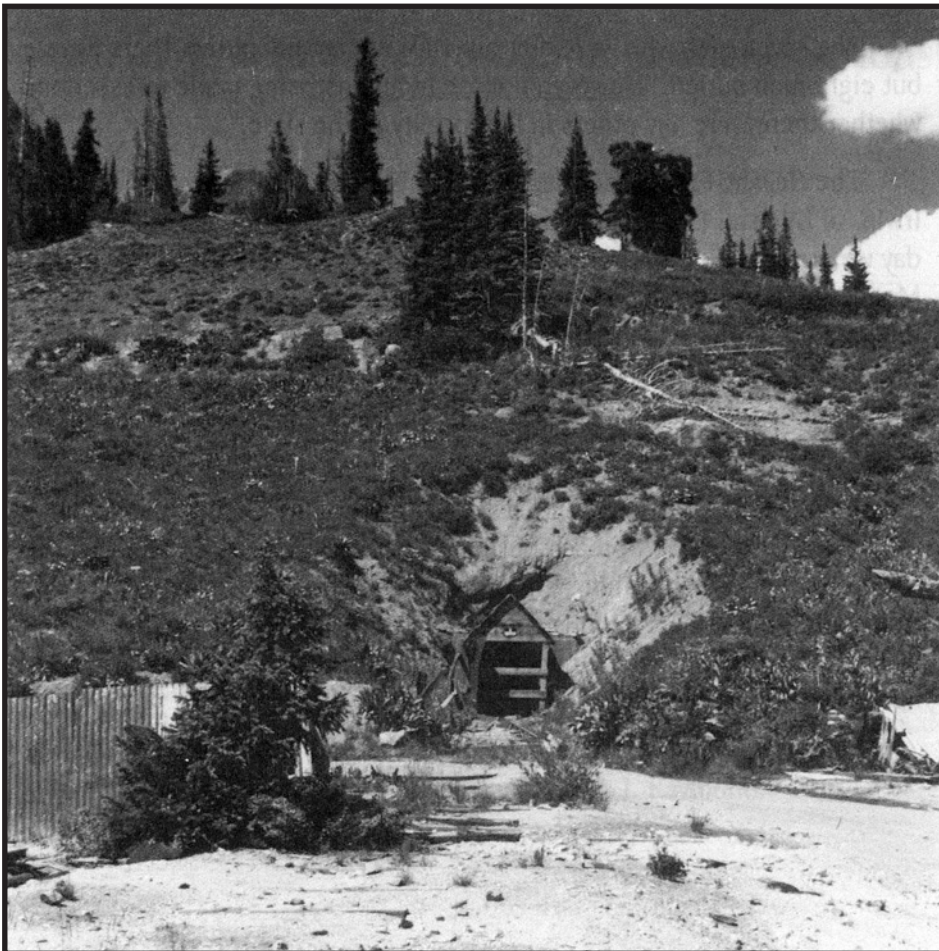
Figure 20. — The Ruby Chief Mine Tunnel as it appeared in August 1981.
