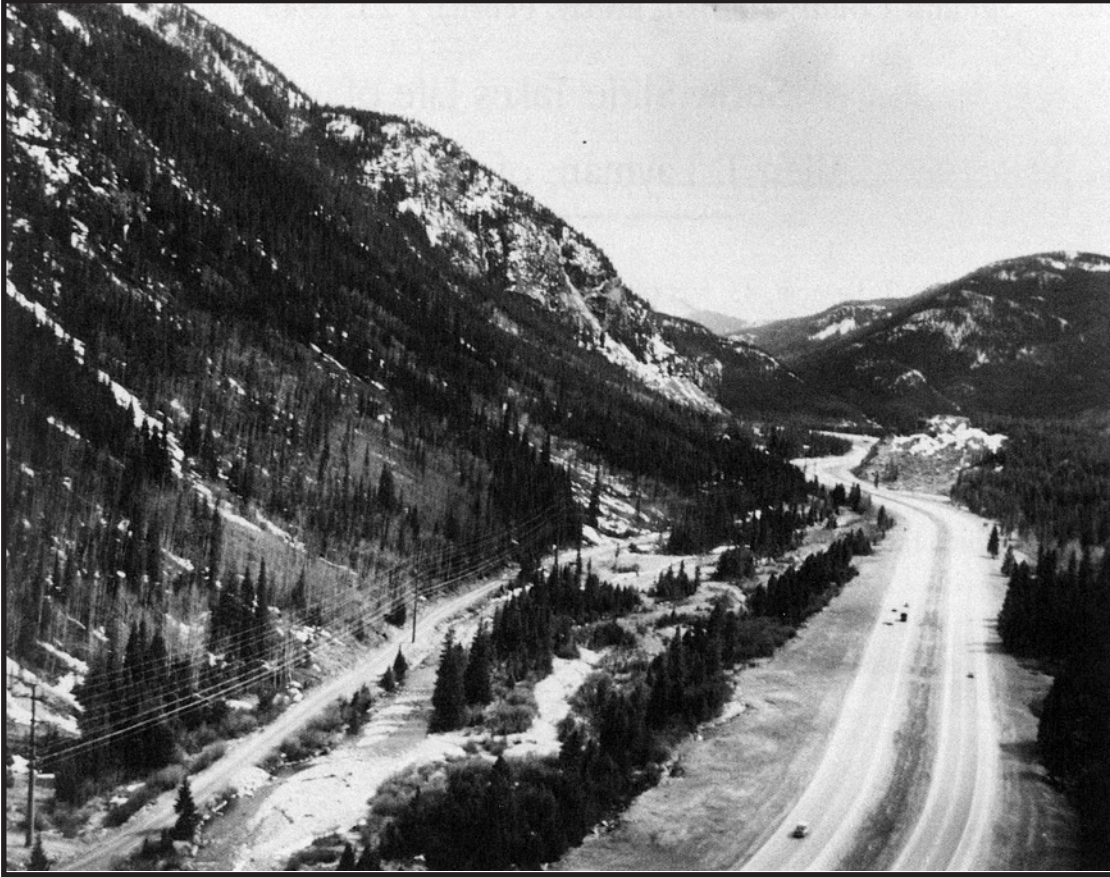
Figure 44. — Looking south up Ten Mile Canyon from the top of the highway cutbank, near Highway Mile Post 199. The old Colorado and Southern Railroad grade (left of the stream) is now a paved bicycle path. Mile Post 122 on the Colorado and Southern Railroad and Curtin (Uneva Lake) were just left of the lower left corner of this picture. Railroad Mile Post 123 was close to the place where the two lanes of Interstate 70 curve to the right (June, 1981).
