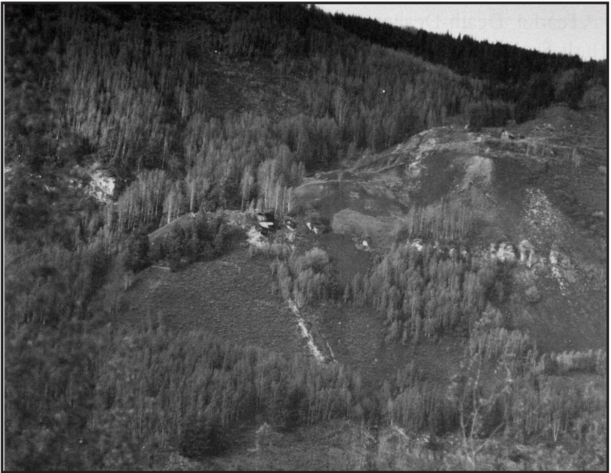
Figure 21. — Smith-Hill anthracite coal mine on the southwest edge of Anthracite Mesa in the Slate River drainage about 4 miles northwest of Crested Butte, June 1981. Six men were killed and 21 injured by an avalanche at this site on January 31, 1883.
