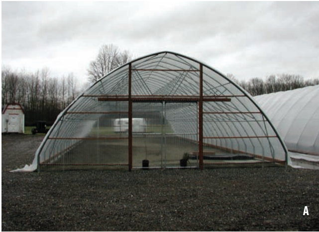
Figure 4.10 —(A) Greenhouses are covered with transparent coverings such as plastic sheeting or (B) hard plastic panels to maximize the amount of sunlight reaching the crop. Photo A by Tara Luna, B by Thomas D. Landis.
