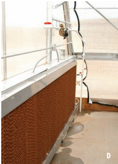
Figure 4.15 —(A) Fully controlled greenhouses contain heating and cooling systems and sophisticated controllers. (B) Greenhouses heat up quickly during sunny weather and must be designed for cooling with interior circulation fans and (C) exhaust fans and vents. (D) In dry climates, fans pull air through wet walls, where it is cooled by evaporation. (E) A quick application of irrigation water can also be used to cool crops. Photo A by Jeremy R. Pinto, B-E by Thomas D. Landis.
