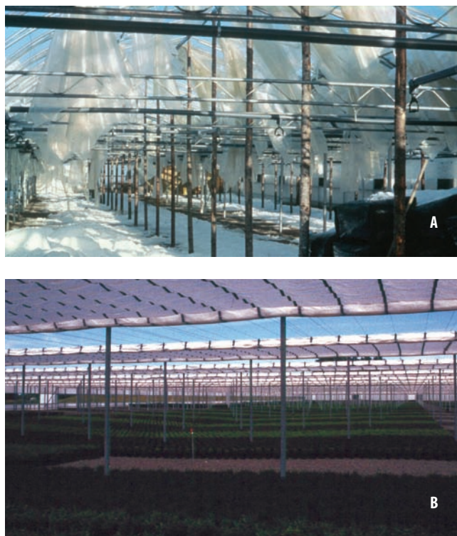
Figure 13.10 —(A) Fully enclosed greenhouses can be used for overwintering sensitive species but snow removal is necessary in cold climates to prevent damage. (B) Retractable-roof greenhouses are better for overwinter storage because they can be opened to allow snow to cover plants. Photos by Thomas D. Landis.
