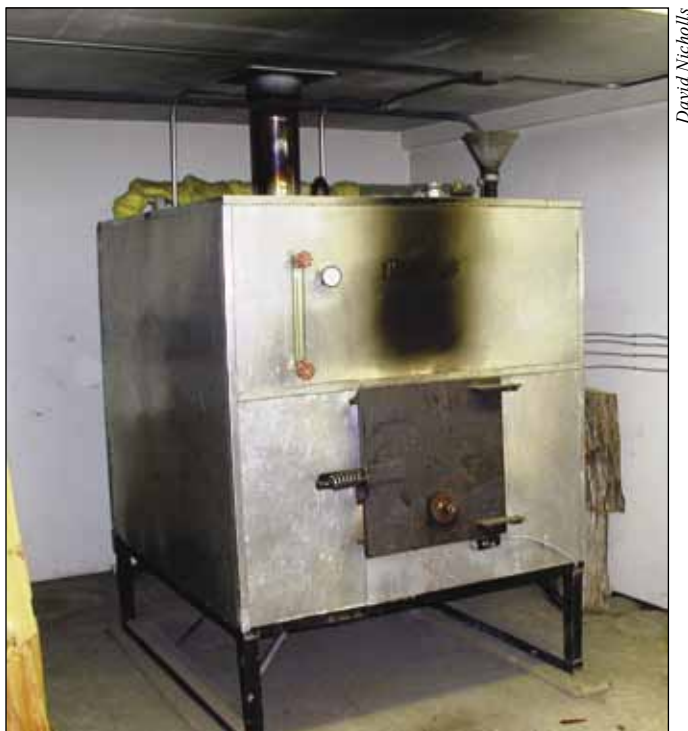
Figure 3—Original wood energy combustion system, in operation from 2001 to 2006, at St. Nick Forest Products (formerly W.R. Jones and Son Lumber Co.).
