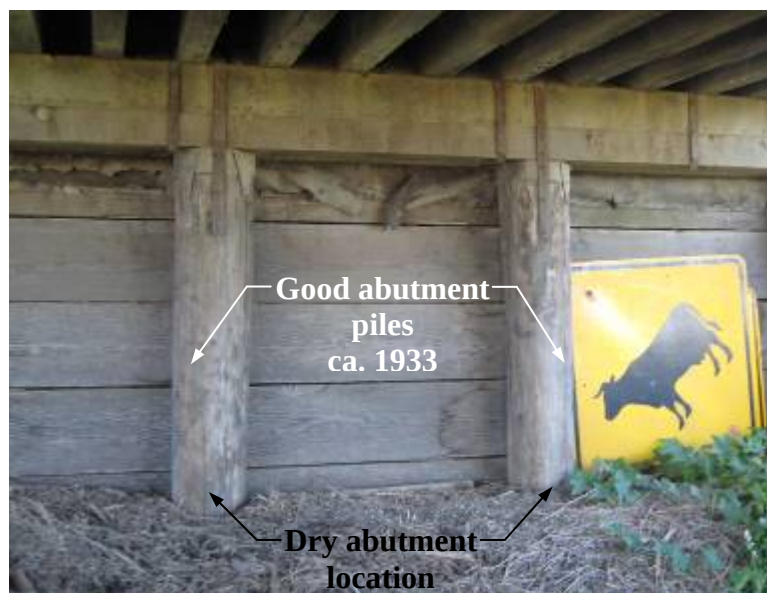
Figure 4-1. Good piles kept above and back from stream channel lasted longer than other pile locations
