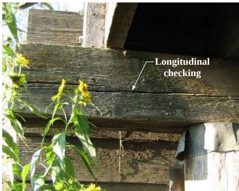
Figure 4-13. Members must be properly seasoned prior to treatment to avoid unwanted checking and associated deterioration
