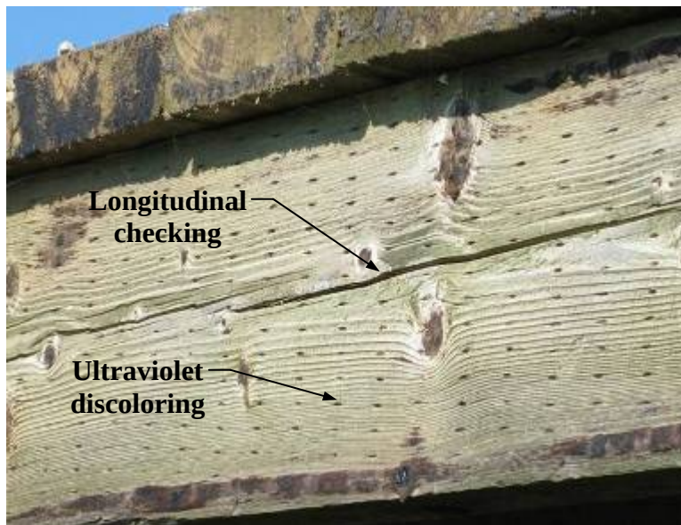
Figure 4-21. Typical checking seen on exterior stringers due to seasoning and direct sunlight
