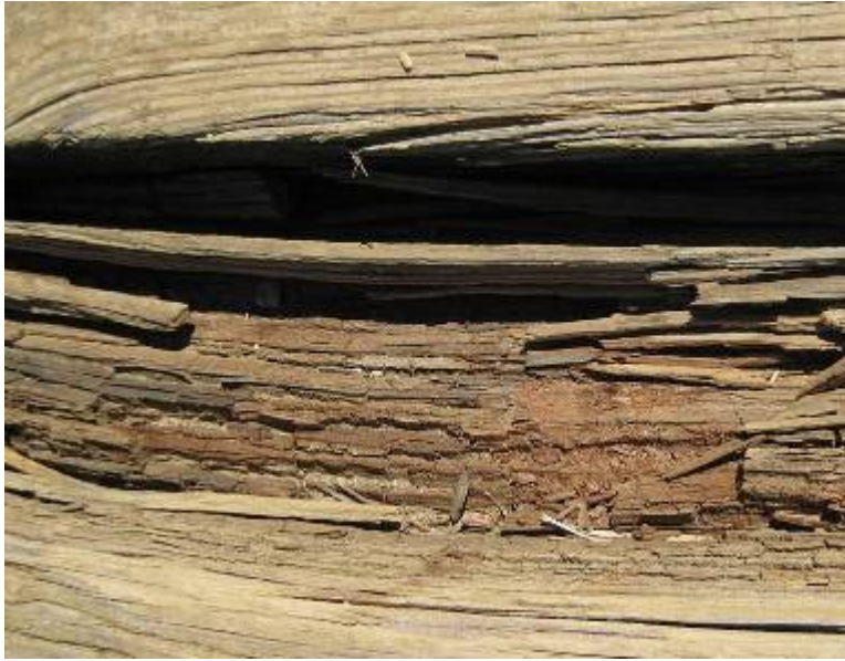
Figure 4-27. Pooling water allowed brown rot to grow on mechanically damaged deck surface
