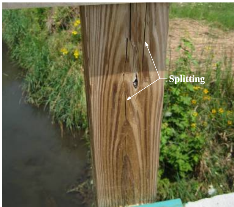
Figure 4-61. ACQ railing post with splitting that is generally associated with waterborne treatments
