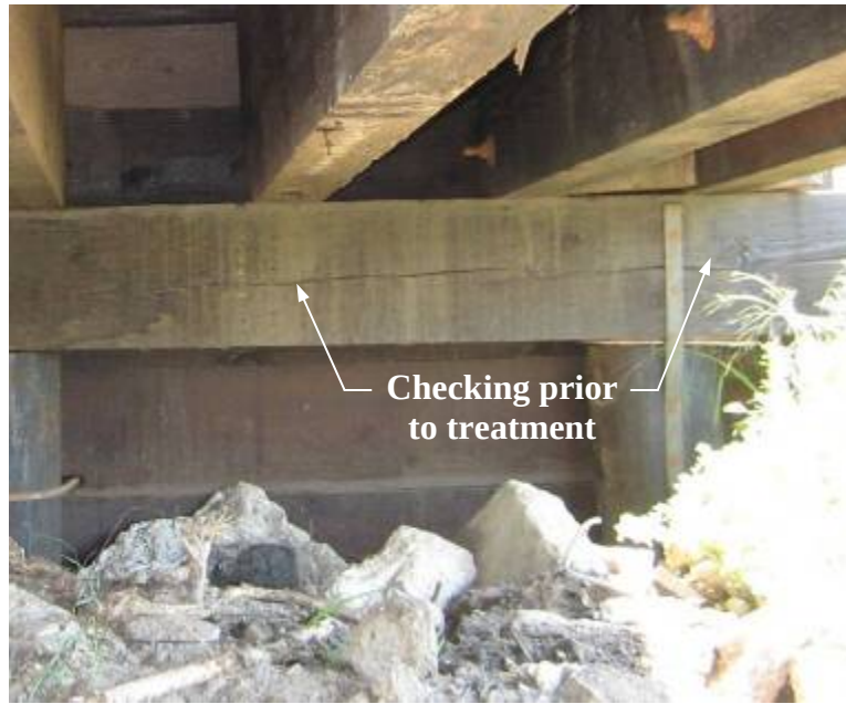
Figure 4-31. Good cap beam with seasoning prior to treatment allowing preservative to infiltrate longitudinal checks creating a complete preservative barrier
