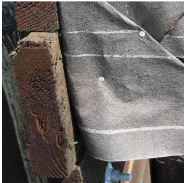
Figure 4-48. Good end grain treatment
