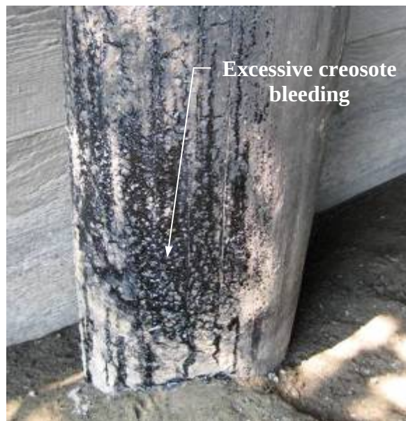
Figure 4-5. Creosote bleeding on the sun exposed side of pile can be minimized by vacuum, steaming, or expansion bath during post-treatment process
