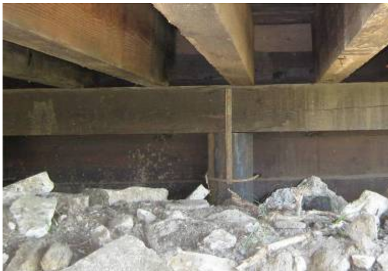
Figure 4-34. Backwall with good in-service condition kept high and away from stream channel
