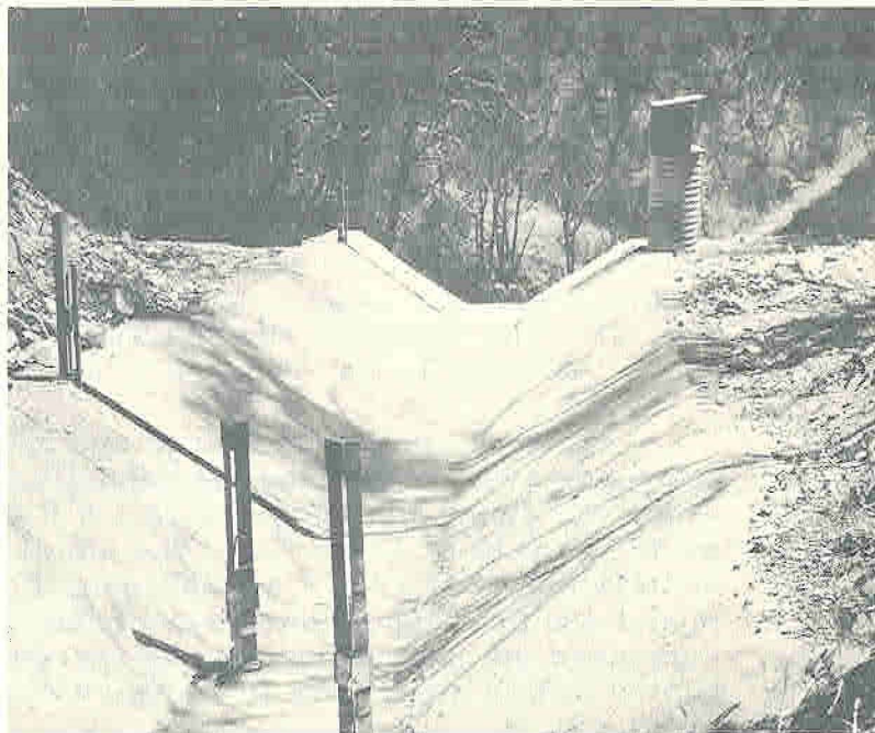
Figure 1.--Typical large flume installation showing approach condition, instrumentation, construction, and free overfall.
