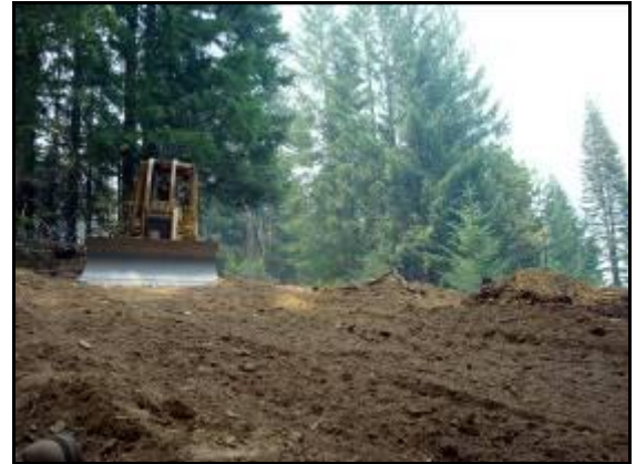
Photo courtesy Redding Hotshots A bulldozer July 5, 2008 on the Lime Complex.
