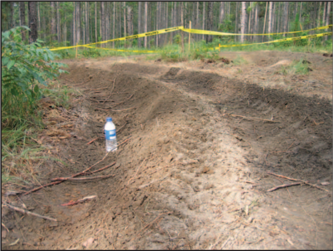
Figure 54—Loop B, 8-inch rut on the turn.
