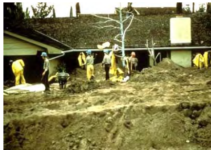
Figure 1 —Post fire erosion problem.
