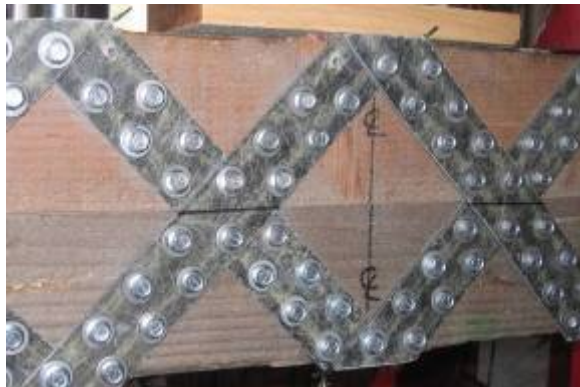
FIGURE 2. TWO MEMBERS STACKED AND FASTENED WITH FRP STRIPS AND SCREWS.
