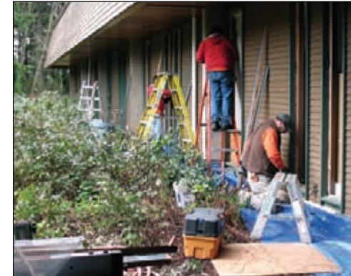
Contractor installs energy-efficient windows at Olympia Lab.
