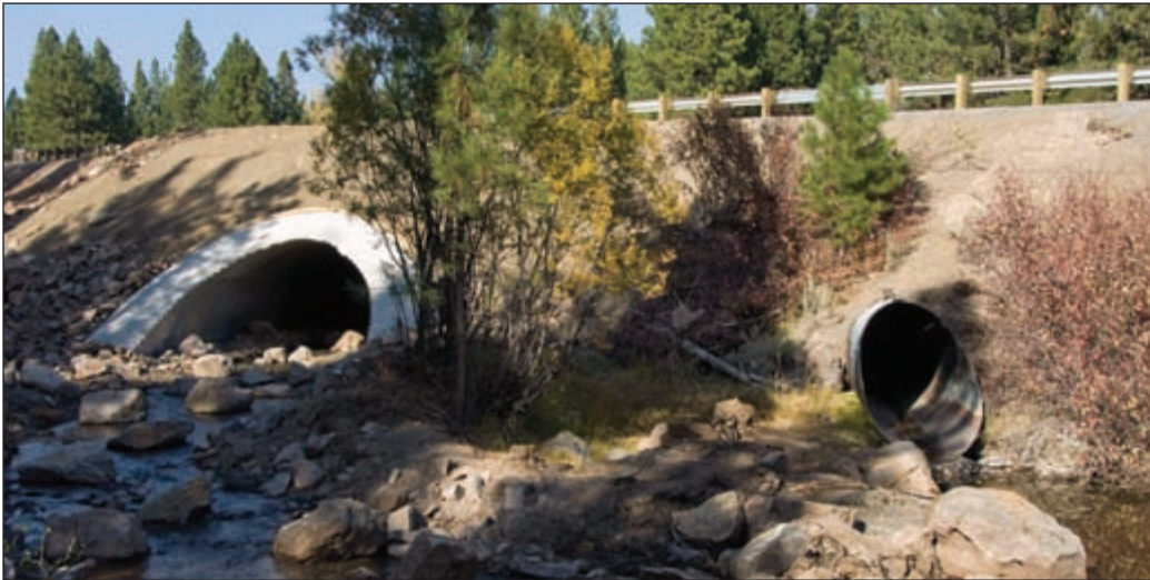
The new culvert on the left was designed to improve passage for aquatic organisms. The old culvert is on the right.
