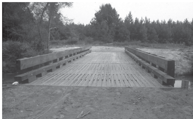
FIGURE 1 Spirit Creek Bridge at time of construction (1991).
