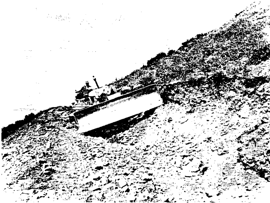
Figure 5.--B. After the platform is constructed, the upper two feet of the steep vertical cutbank are knocked down to aid in backsloping.
