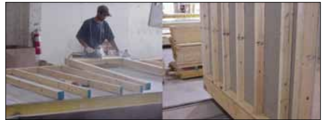
Figure F4. Wall construction (left), and use of predrilled spruce-pine-fir (SPF) wall studs (right).
