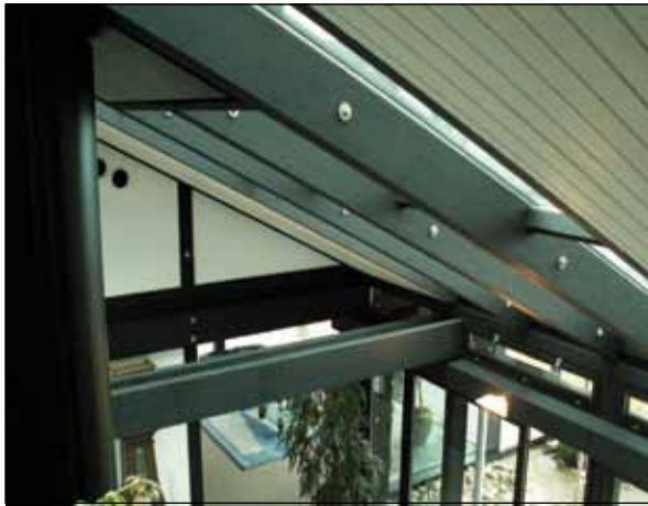
Figure GB1. Painted laminated beams are used throughout Plant GB homes.
