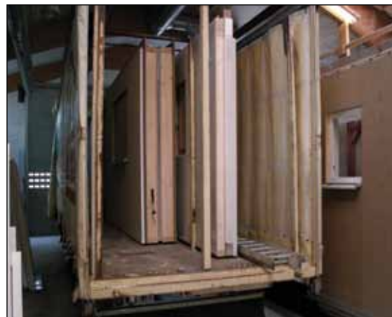
Figure GF7. Wall components loaded onto truck for delivery to building site.
