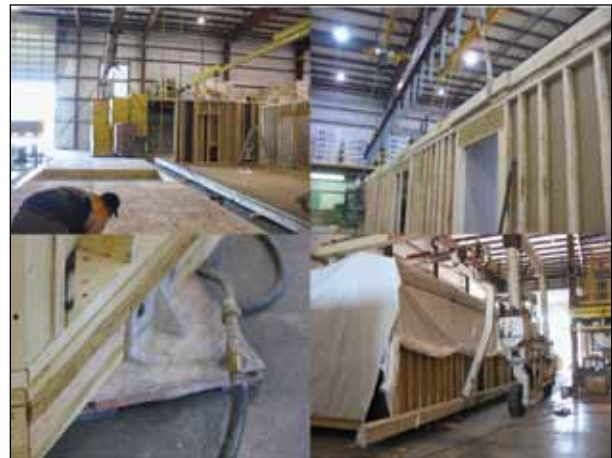
Figure B4. Walls and floors are moved with overhead cranes (top left and top right); modules in process are moved using pneumatic air pads (bottom left); completed modules are loaded onto trailer for delivery using boat transporter (bottom right).
