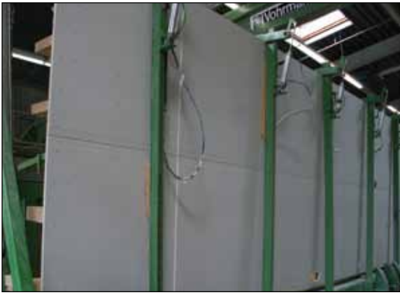
Figure GA18. Butterfly table flips the middle floor construction so other side can be worked on.
