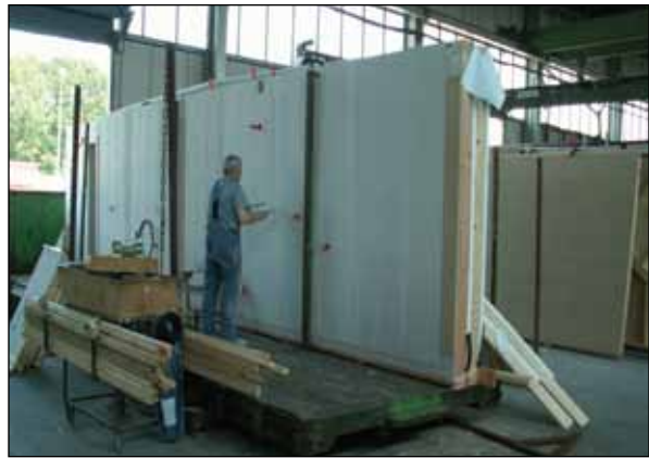
Figure GA22. Finished wall sections are oriented vertically and loaded onto a metal platform, which is placed on truck bed for transport.
