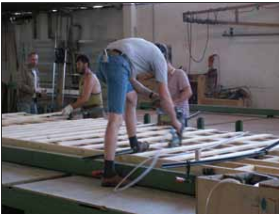
Figure GH3. Ceiling being constructed.
