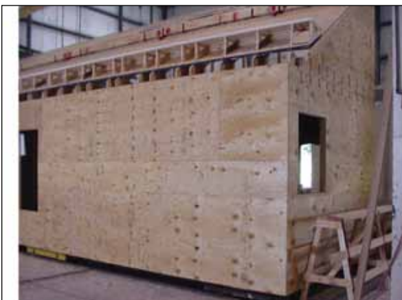
Figure F8. Plant F typically uses 3/8 in. pine plywood wall sheathing.
