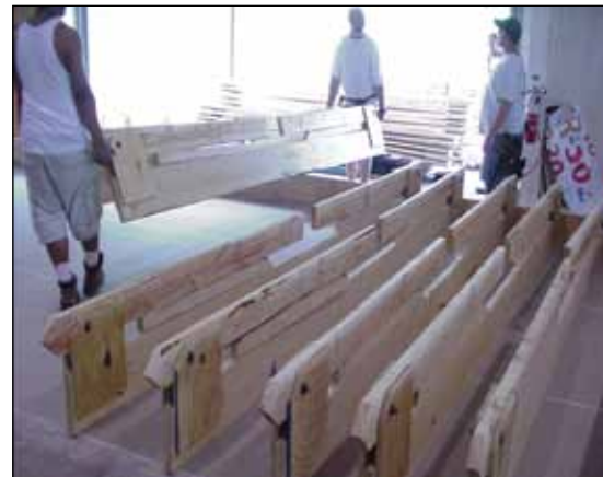
Figure F5. Installing rafters on ceiling drywall.
