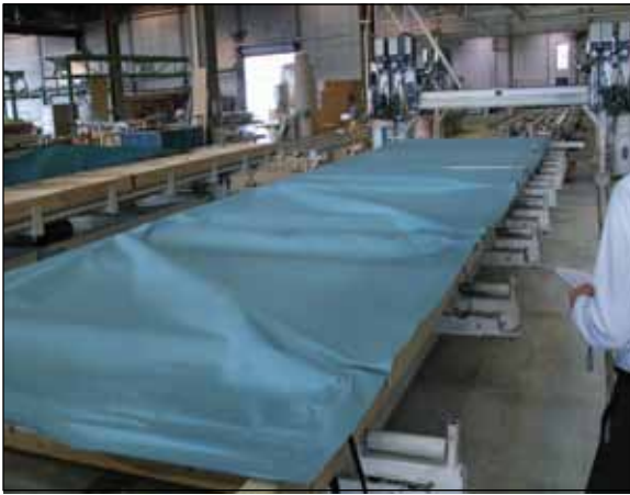
Figure GG8. Paper moisture barrier placed on wall panel section.
