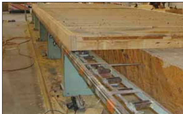
Figure B2. Floor frame constructed on jig table.
