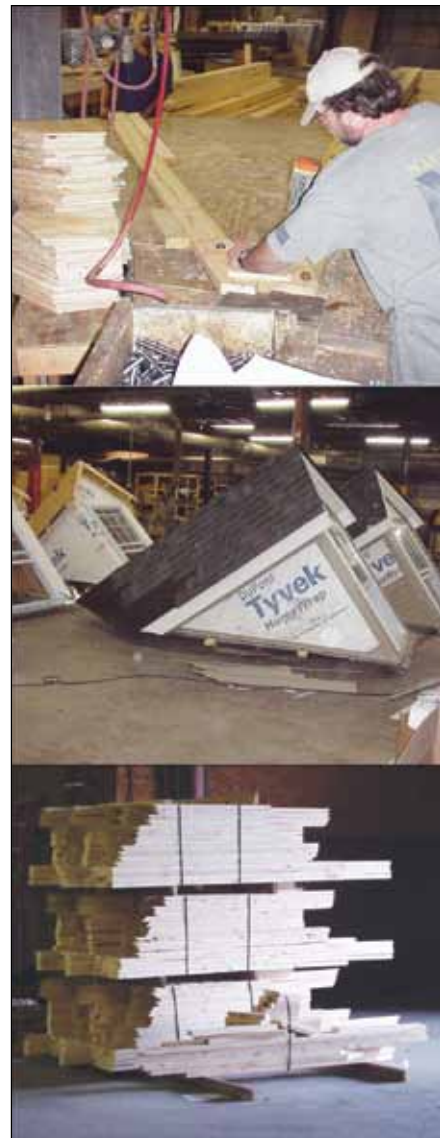
Figure F10. Rafters being built in component plant (top). Constructed dormers (center) and component parts assembled in kits by module (bottom).
