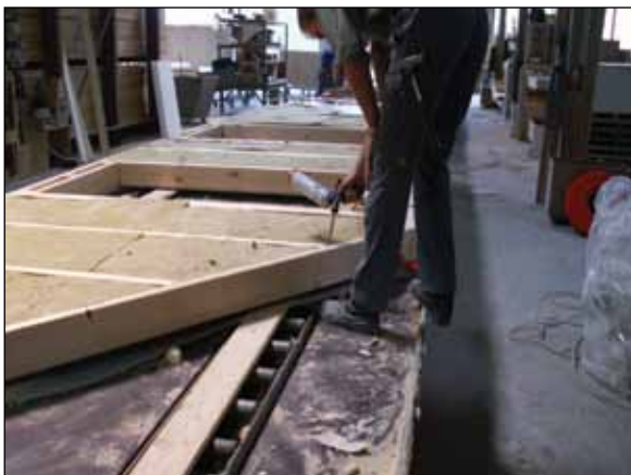
Figure GA14. Expanding foam used to fill voids and completely insulate wall panels.
