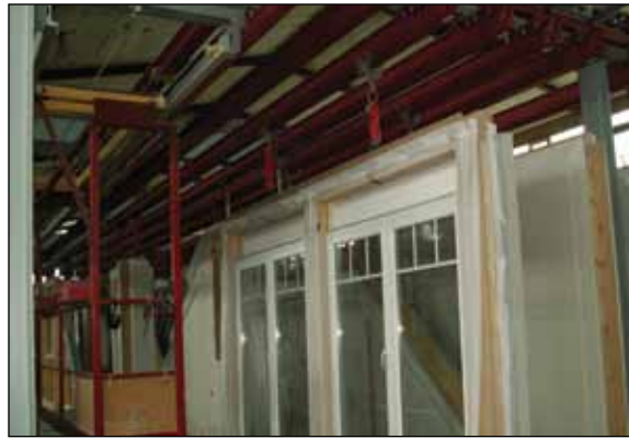
Figure GC8. Elevated cart for worker access to vertical wall.
