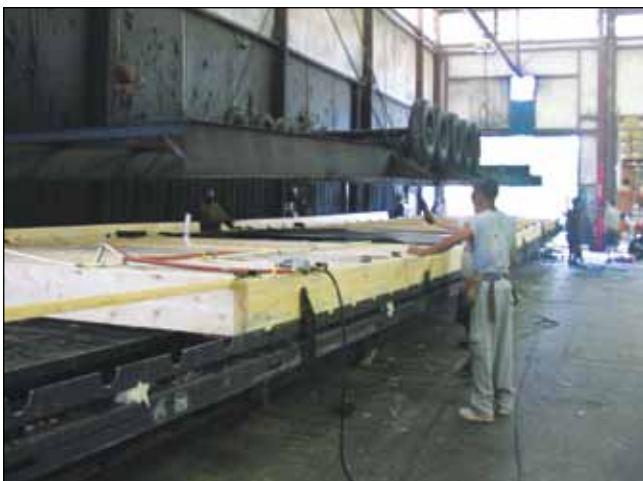
Figure C2. Metal frame with wheels being attached to constructed floor frame.
