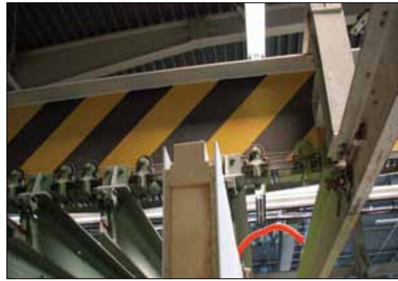
Figure GA15. Top of wall panel shows channel developed for electrical conduit placement.
