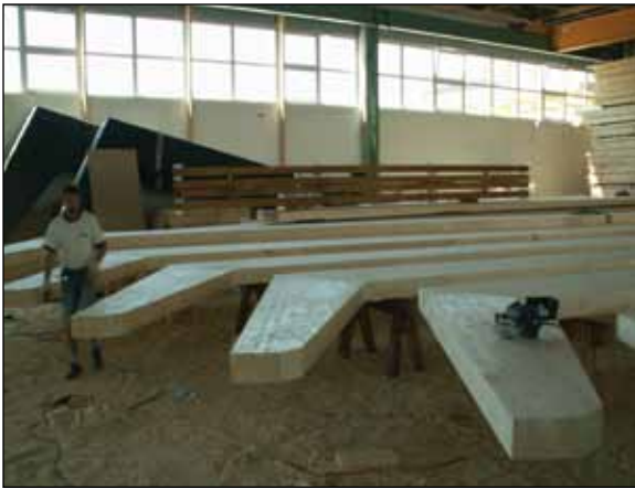
Figure GH1. Laminated beams in process at Plant GH.
