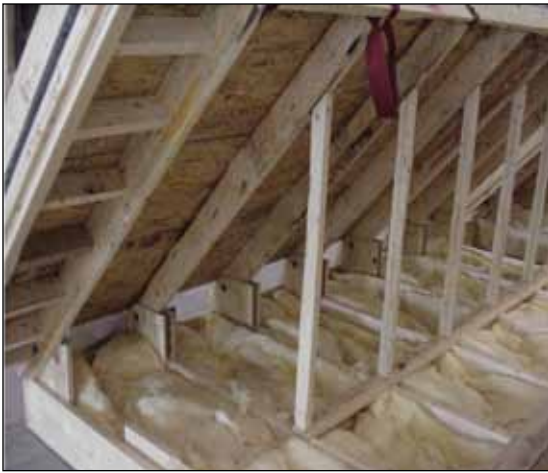
Figure F6. Installed rafters and knee brace in attic module.
