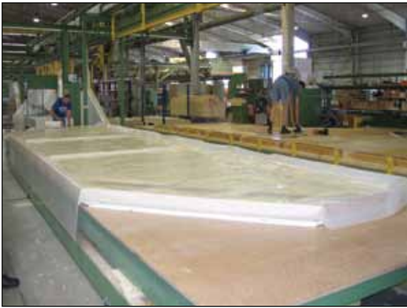
Figure GD5. Plastic moisture barrier installed over wall panel.
