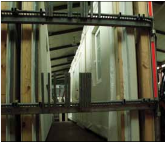
Figure GC12. Wall components are fastened in a rack on the transport trailer.
