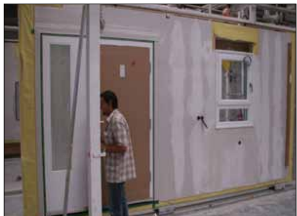
Figure GE10. Note electrical conduits, interior window shade, and installed doors and windows.
