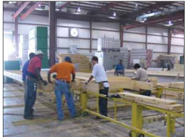
Figure A4. Floor being assembled on non-functioning adjustable jig. These men are constructing a floor section on a floor jig, the metal framework that the wood floor is resting on. Wheels on the jig base allow the overall frame to move.
