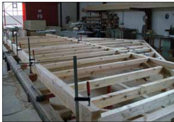
Figure GC9. Gable walls are built one on top of the other to ensure symmetry.
