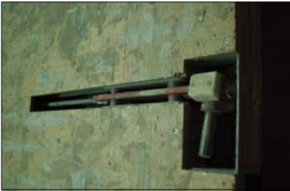
Figure GC5. Specialized wall table clamp that can retract into table to remove trip hazard.
