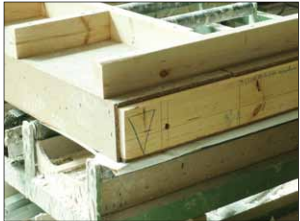
Figure GH10. Sawyer marks component placement on bottom plate.
