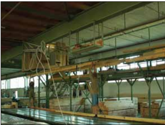
Figure GH9. Wall components are cut in upstairs mezzanine and carpenters reach for them.
