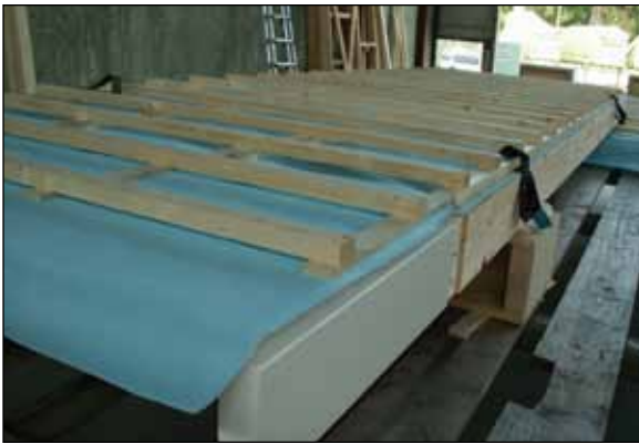
Figure GA19. Roof table showing furring strips for tile shingles (installed on site), blue plastic water proofing, and painted exposed joist.
