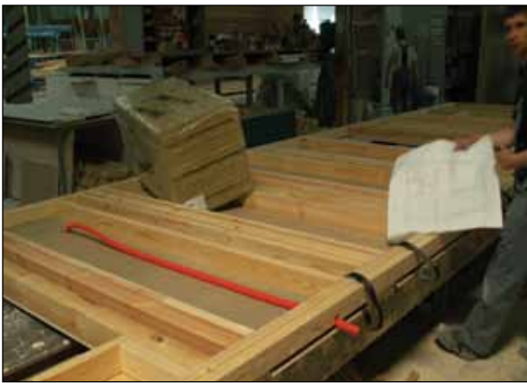
Figure GA13. Framed and drywalled wall showing bats of mineral wool and plastic electrical conduit.
