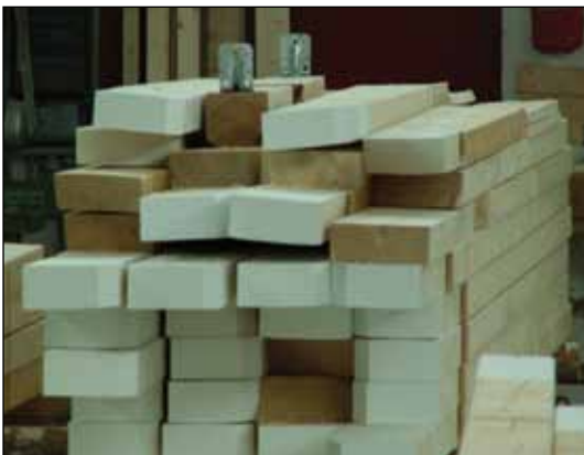
Figure GC13. Roof rafters are cut and painted at the factory but assembled on-site.
