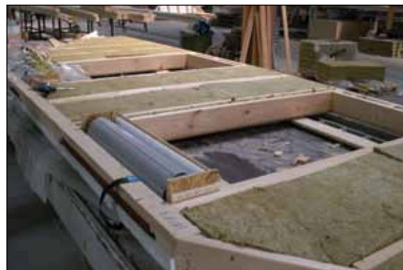
Figure GA11. Timber frame showing red electrical conduits, mineral wool insulation, and exterior window shade.
