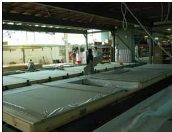
Figure GH12. Other side of wall panel has moisture barrier and sheathing attached.
