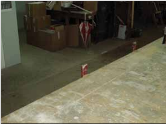
Figure GC6. Stop bracket on wall table used to position wall frame elements.
