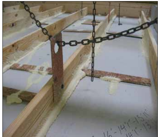
Figure C9. This ceiling (middle floor) section shows adhesive foam used to attach drywall to ceiling joists. Note the metal bracket and chain used by a crane to hoist the ceiling section.
