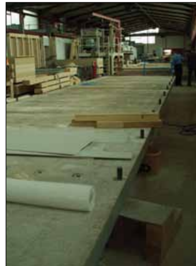
Figure GC4. Wall-build table showing stops used to position wall-frame elements.
