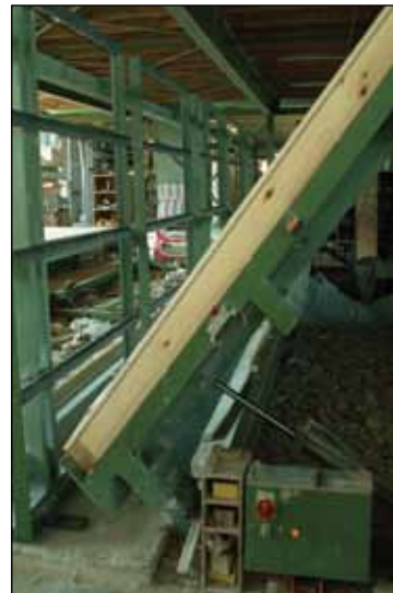
Figure GH11. Butterfly table flips wall section after one side is sheathed.
