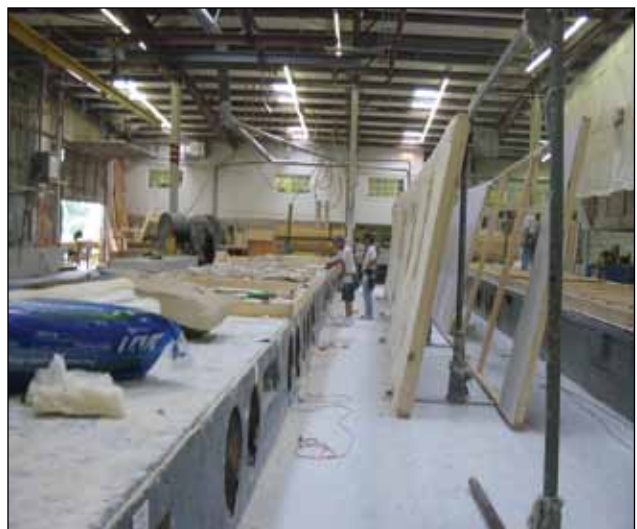
Figure C5. Long wall tables with completed walls standing to the side.
