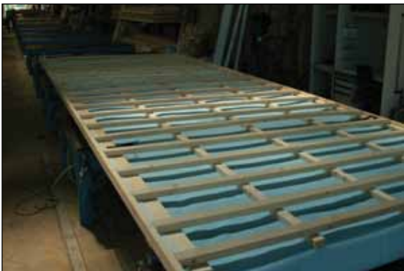
Figure GA20. Roof table showing furring strips and sheet of plastic water proofing.
