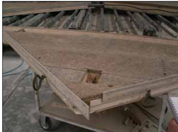
Figure GE8. Troublesome components, such as this gable, can be pulled offline. Note eyehooks used for vertical hanging.
