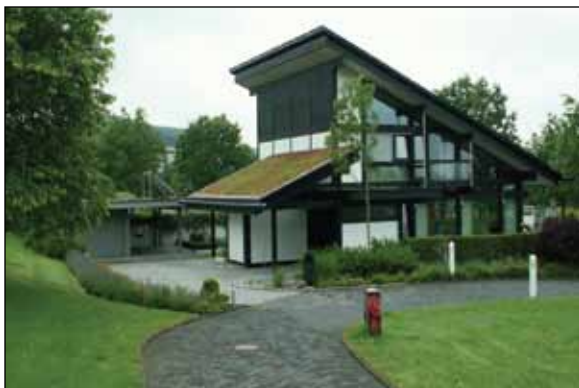
Figure GB3. Plant GB model home located on site.
