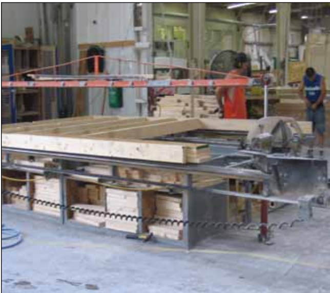
Figure C7. An adjustable carriage was used to select the angle required to saw the wall for angled ceilings.
