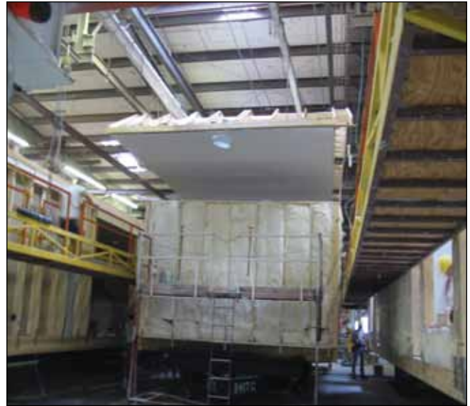
Figure C8. Roofs constructed in the upstairs loft were moved by overhead cranes.
