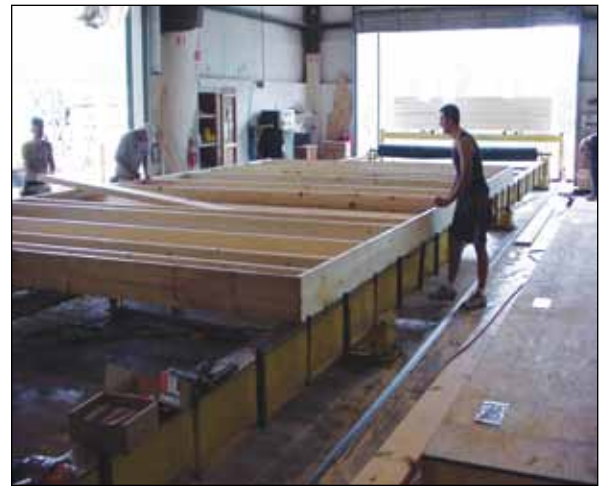
Figure F3. Joists installed at floor framing table.
