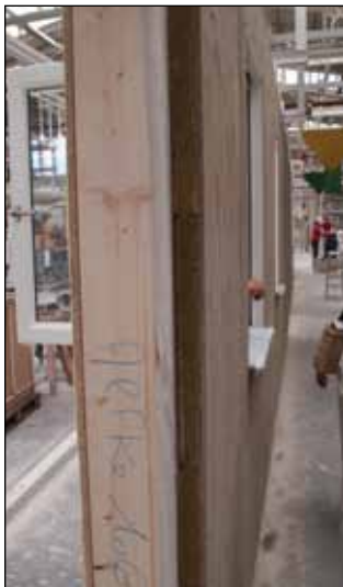
Figure GE7. Detail showing many layers of the exterior wall.
