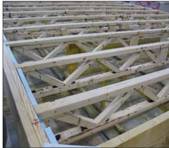
Figure A3. Floor made with Open Joist 2000.
