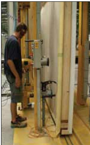
Figure GD6. The HELO TEC machine bored holes in walls for electrical switches and outlets.
