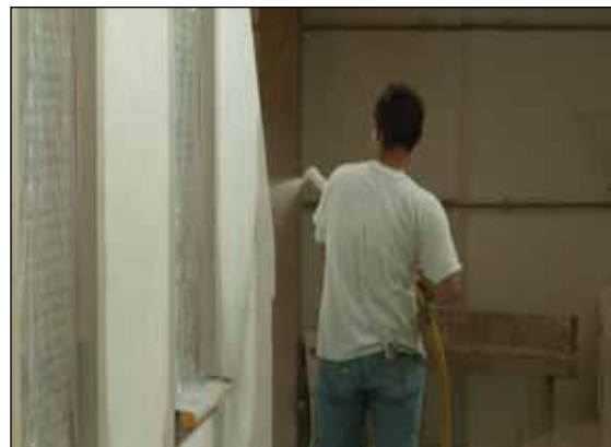
Figure GF8. Stucco being sprayed onto wall panels using fiberglass mesh.
