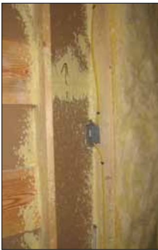
Figure A7. Foam spray sealing drywall gaps from rear and adhering to studs.
