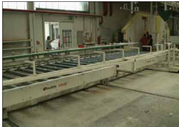
Figure GE9. Butterfly transfer table raises wall panel for vertical hanging onto line (to right).
