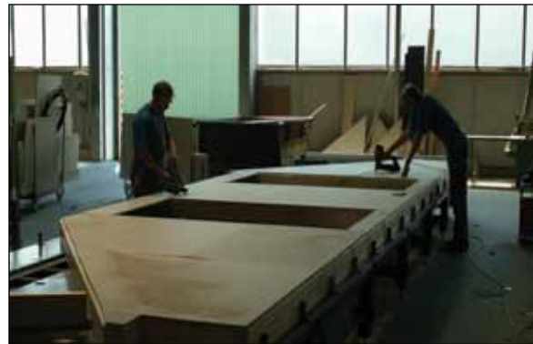
Figure GA10. Nailing sheathing to the timber frame at the wall table station.
