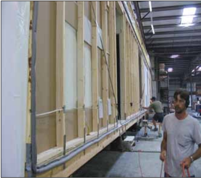
Figure C6. Marriage wall characterized by lack of insulation and a gasket seal. Note the small drywall panels providing additional support.
