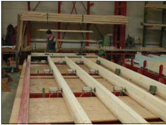
Figure GF9. Roof table using pneumatic jigs to place and hold rafters.
