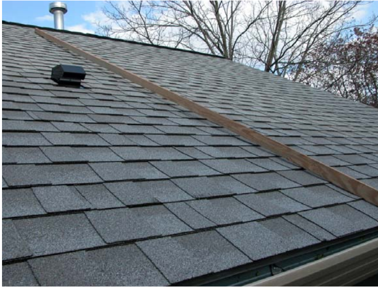
Figure 1. Noticeable sag of rafters on a single-story home of modest size, constructed in 1940. At the time of construction, regional building codes had not been developed.
