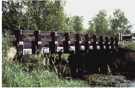
Figure 8. Ciphers stress-laminated deck bridge located in northern Minnesota.
