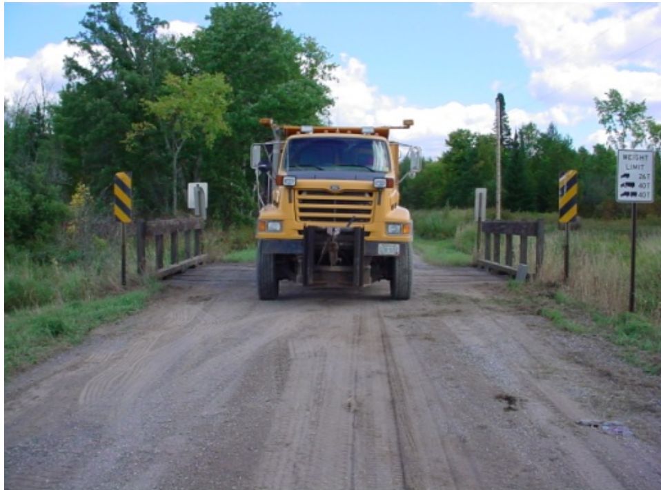
Figure 3.4. Truck positioned on bridge.
