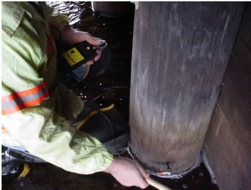
Figure 3.1. Fakopp microsecond timer being used on a timber pile.
