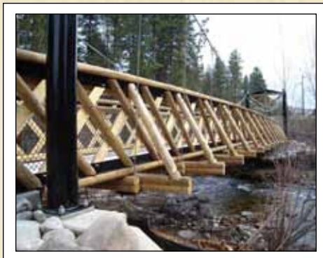
The Rattlesnake Creek bridge near Missoula, Montana, was built using 6-inch-diameter lodgepole pine from a forest in Idaho to demonstrate the effective use of trees killed by the pine bark beetle.
