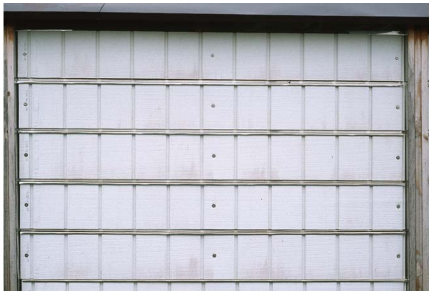
Figure 10. Painted plywood with Z-flashing between panels.
