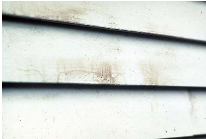
Figure 13. Diffuse extractives bleed on painted boards.
