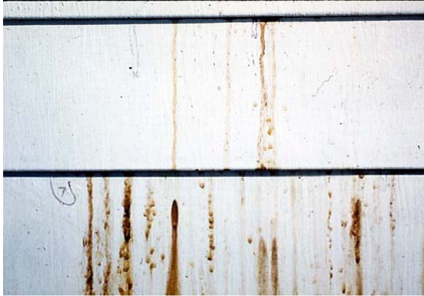
Figure 14. Run-down extractives bleed on painted boards.
