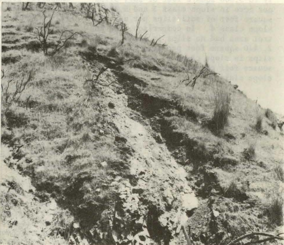
Figure 4.--Soil slippage over underlying rock strata.
