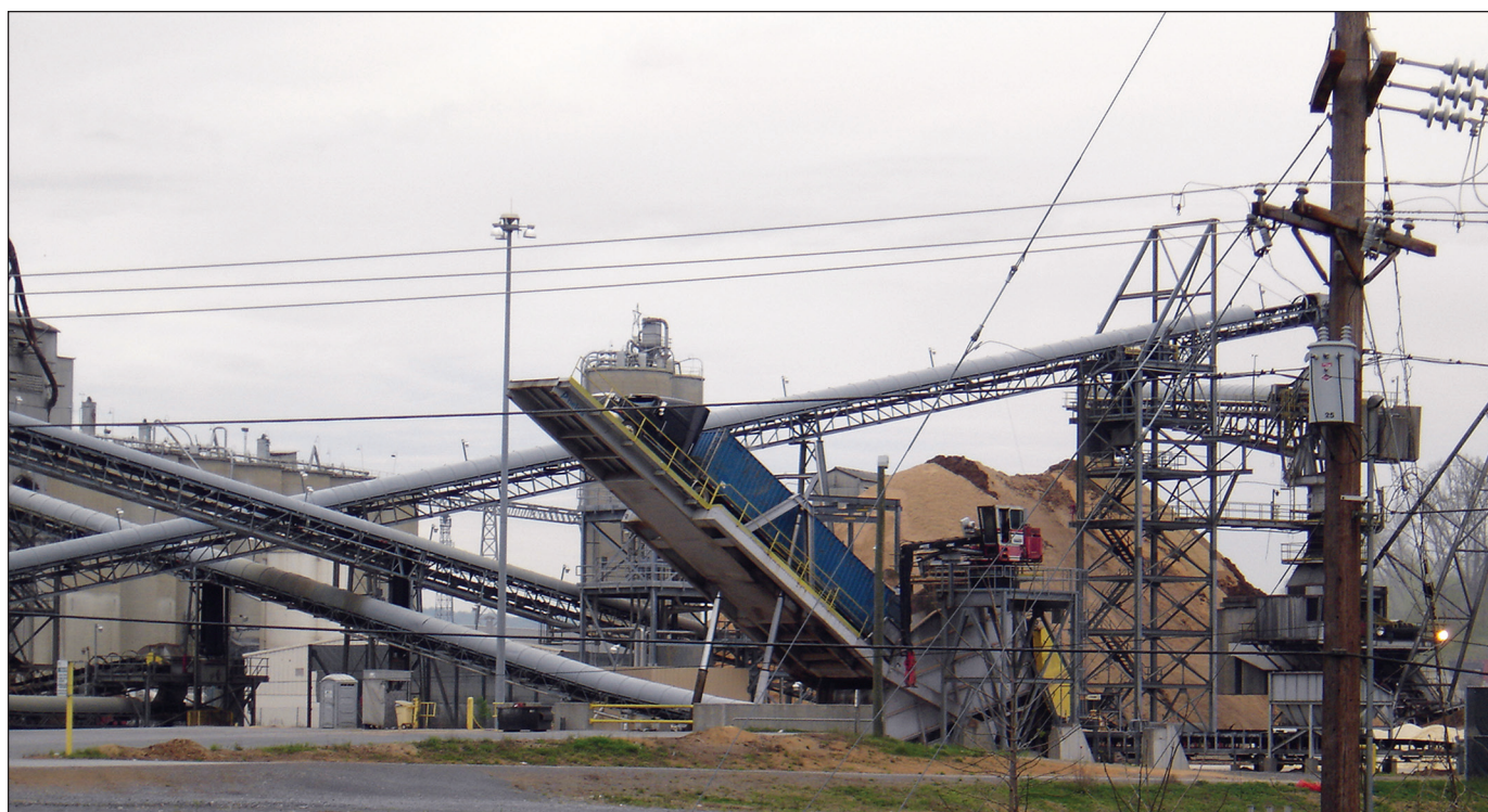
Truck hauling chips, being off-loaded, Kingsport, Tennessee. (photo by Angie Rowe)
