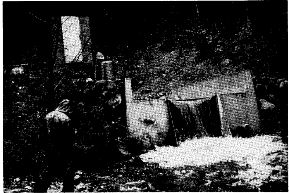
A weir at flood stage at the Hubbard Brook Experimental Forest. Weirs or streamgauging stations like this are used to obtain continuous measurements of streamflow. They are a basic tool for watershed research
