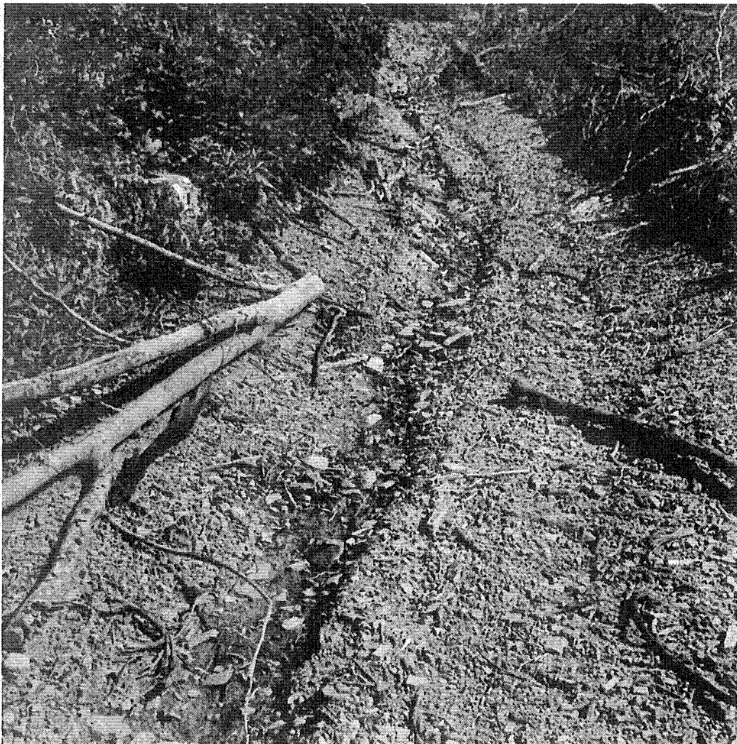
Figure 16.—A steep, gullied skidroad in the Commercial Clearcut Watershed soon after completion of the logging operation.
