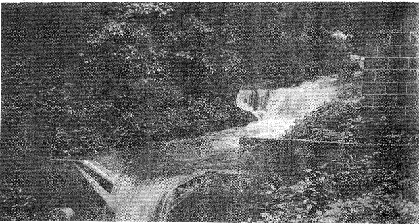
Figure 4.—A stream-gaging station on one of the experimental watersheds.
