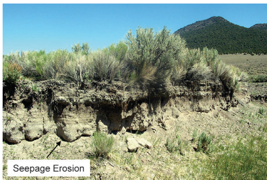
Figure 3.17. Wall of trench located downstream of the headcut shown in fig. 3.16. The eroded “alcove” positioned along the base of the bank was likely caused by groundwater as it emerged from the valley fill. This type of undercutting often leads to bank failure.
