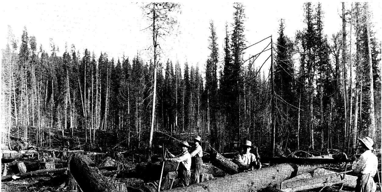
Clearing away debris on Jurgens Flat for experimental plots, 1912.
