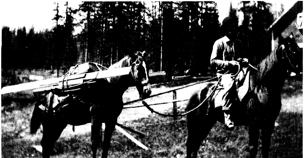
Packing lumber to build a lookout cabin on Experiment Station Lookout, 1917.
