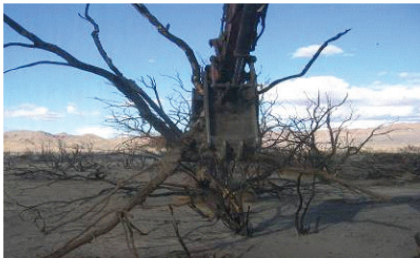
Figure 9. Using an extractor to remove various live and dead trees including saltcedar and Russian olive. From Sisneros (1994).
