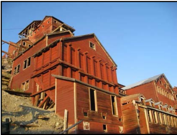
Figure 2: Northwest view of the Concentration Mill Building (June 2009).
