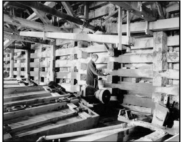
Figure 3: Timber crib foundation wall at level 3 of the Concentration Mill Building during 1976 inspection.
