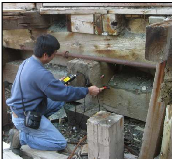
Figure 4: Testing a “header” timber crib member with a stress wave timer device.
