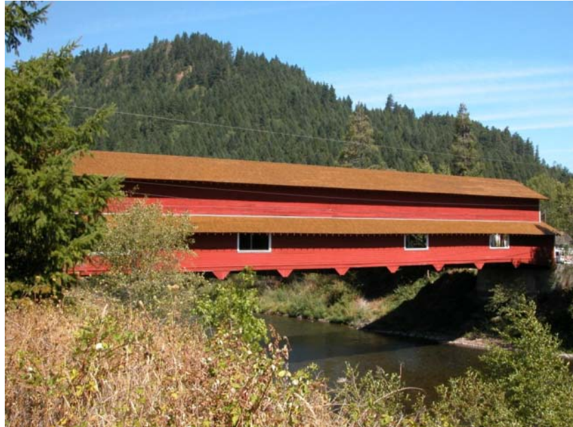
Figure 1. Covered bridge in Oregon.
