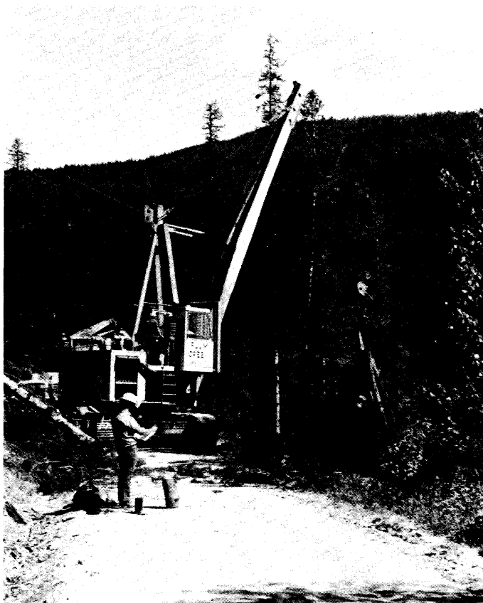
Figure 2.—Yarding with running skyline.
