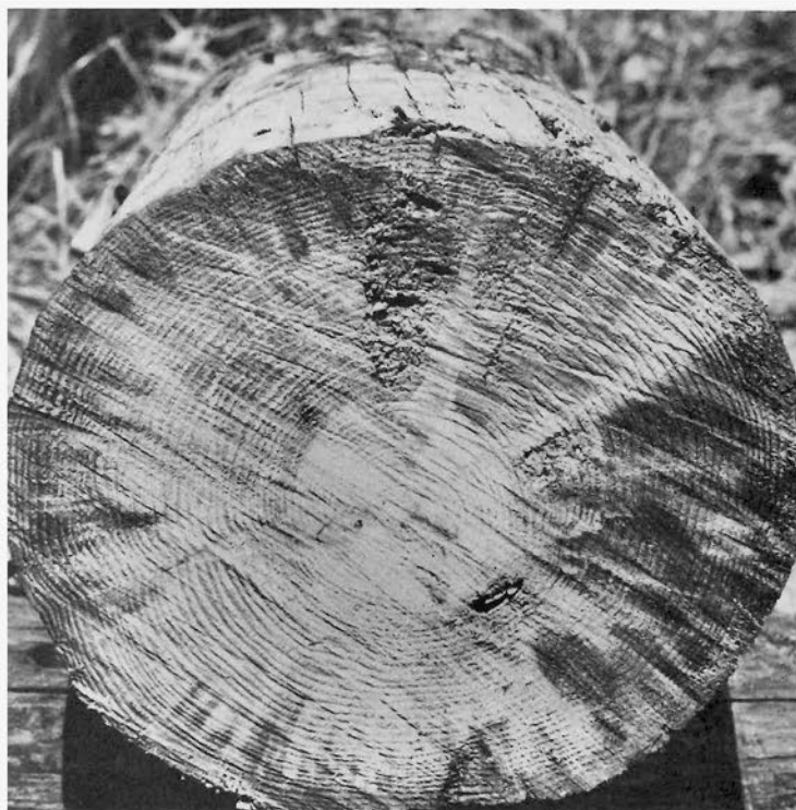
Figure 11.—Wedge pattern of decay.
