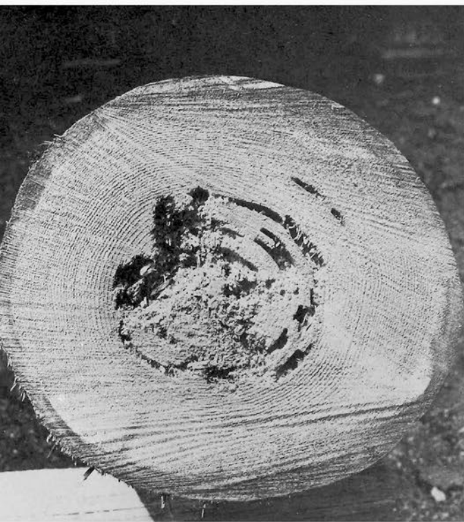
Figure 8A.—Cross section of central decay in cedar.
