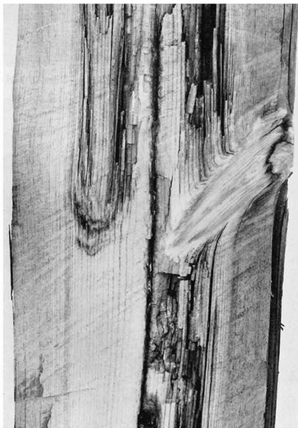
Figure 35.— Large branch stub and associated decay. Note abrupt end to decay column on left. The Shigometer would show an abrupt decrease far beyond the obvious end of the decay column.
