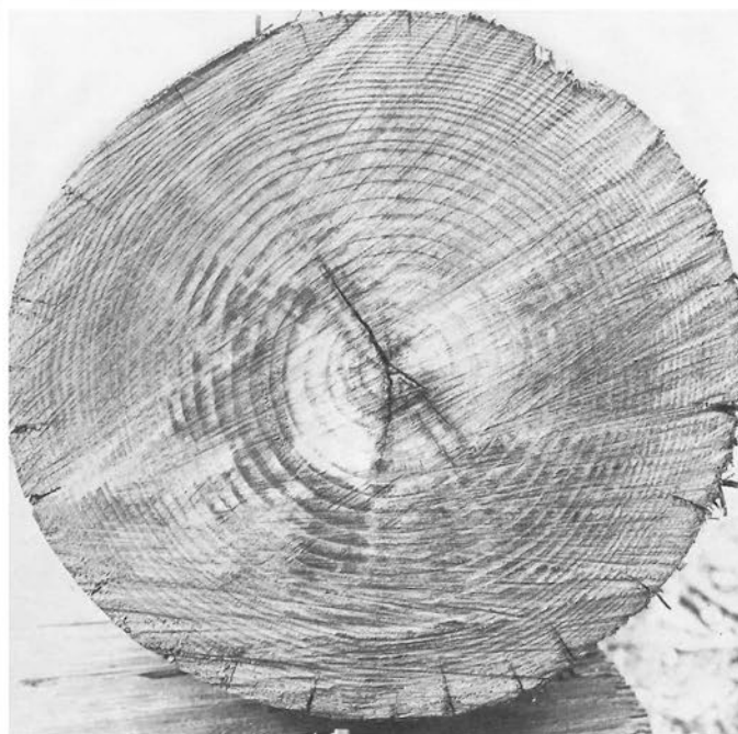
Figure 18.—Beginning stage of in-between pattern of decay. (When used properly the Shigometer will detect this).
