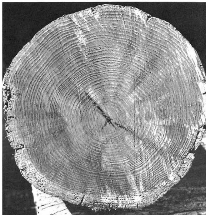
Figure 14.—Soft rot (external decay).
