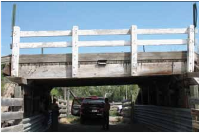
Figure 13. Montana Bridge used for finite element modeling.
