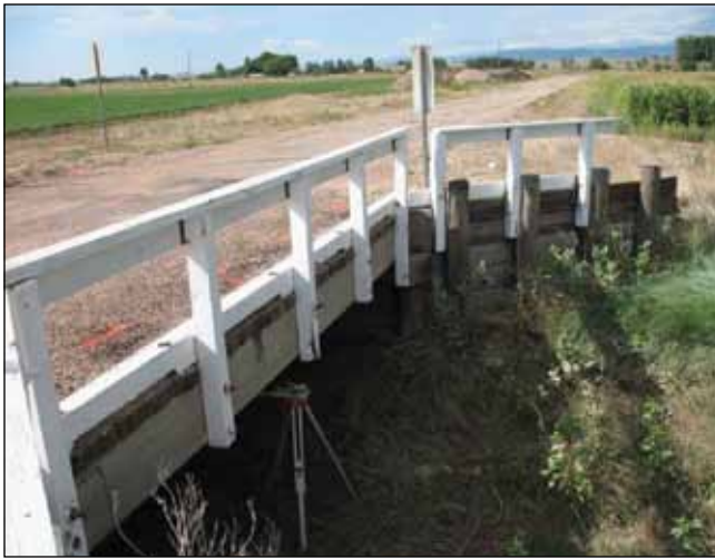
Figure K3. Larimer County Bridge parapet support.
