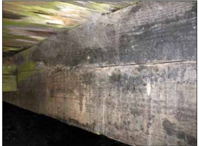
Figure I17. Checking in the girders.
