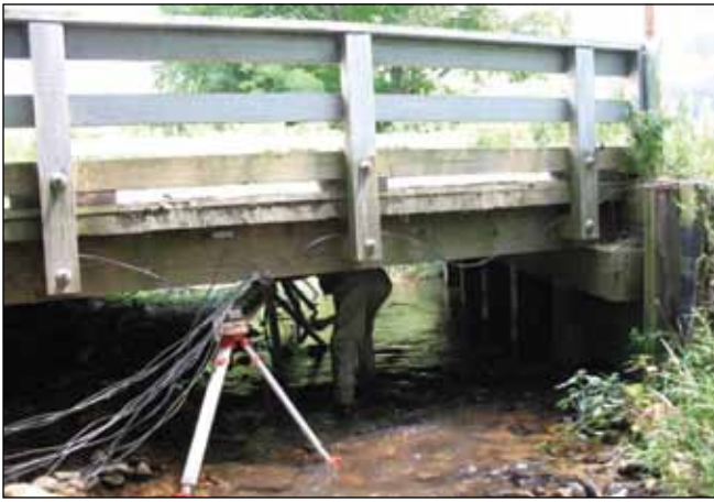
Figure H3. Bald Creek Bridge parapet.
