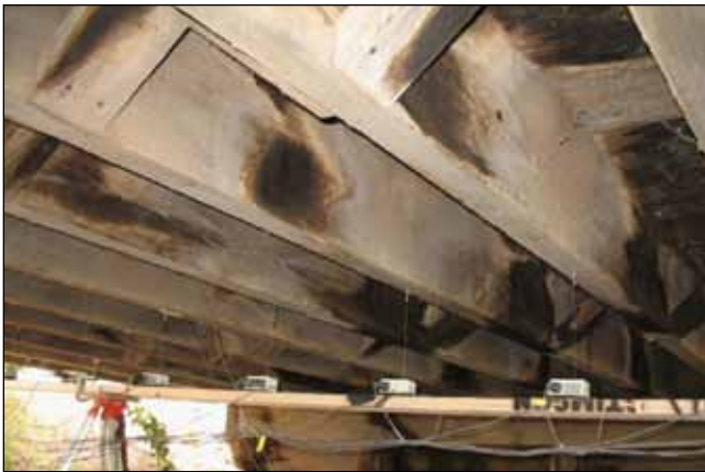
Figure K14. General superstructure condition.
