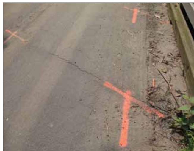
Figure D14. Transition between roadway and bridge.
