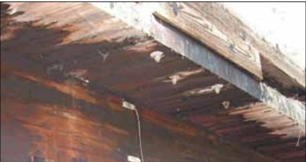
Figure Q14. Washing of creosote at panels ends.
