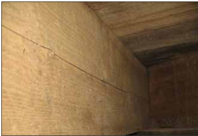
Figure D16. Checking at centerline near abutment.
