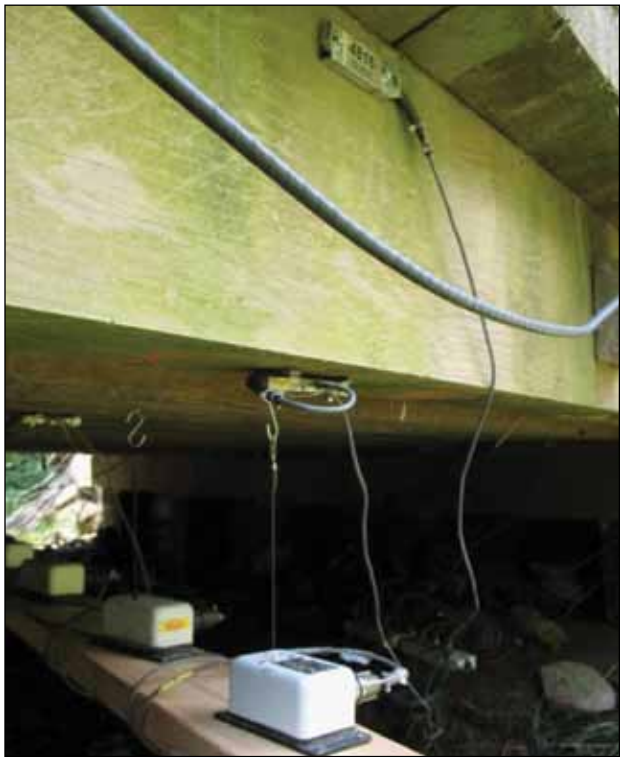
Figure H7. Outside girder strain transducer setup.
