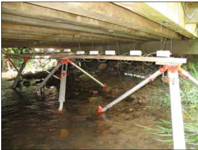
Figure H6. Deflection instrumentation.
