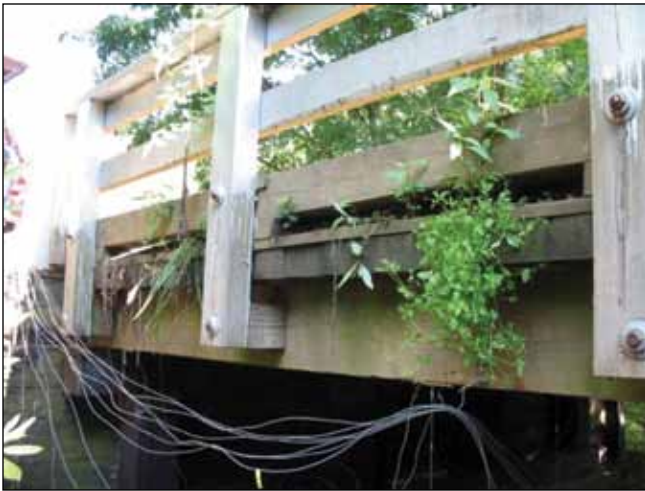
Figure G3. Dix Creek parapet.
