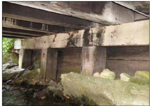
Figure P2. Bridge substructure.
