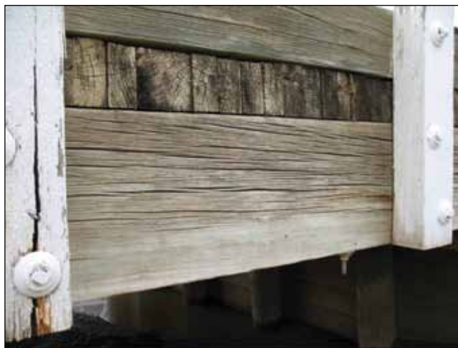
Figure M14. Checking in exterior girders.
