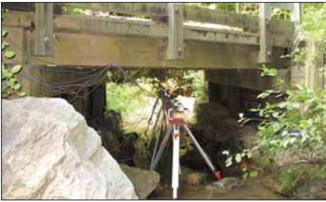
Figure D3. Madison County parapet.
