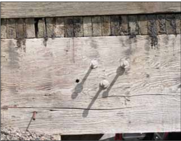
Figure O14. Checking in exterior girders.
