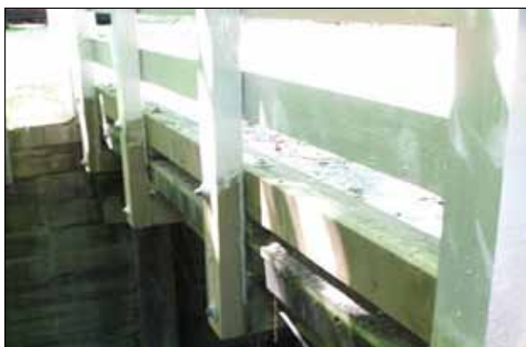
Figure C2. Chestnut Cove Creek parapet support.
