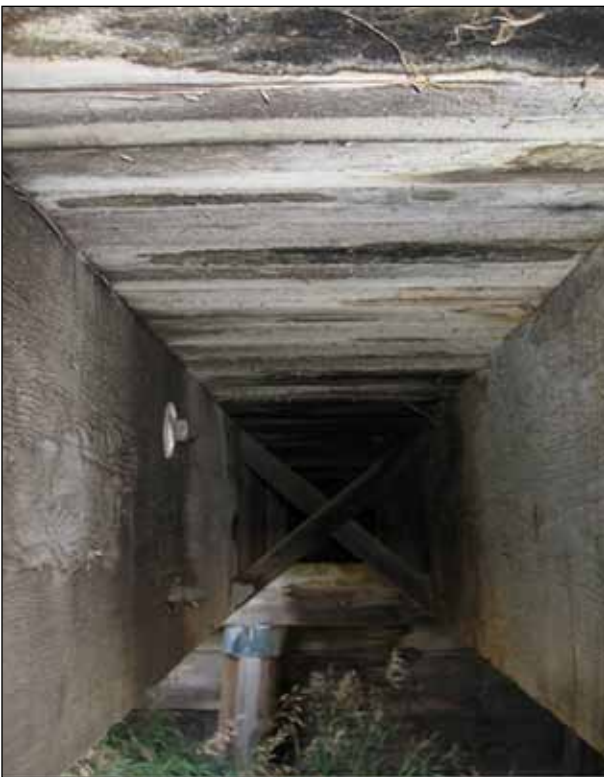
Figure N14. White residue formation on deck.
