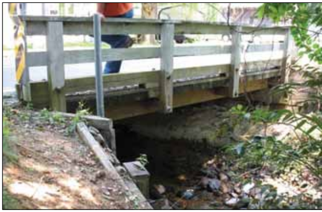
Figure J3. McDowell County Bridge parapet support.
