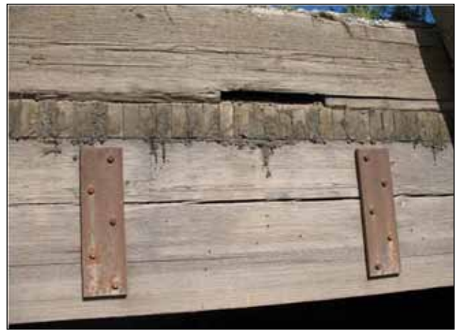
Figure N15. Checking in exterior girders.
