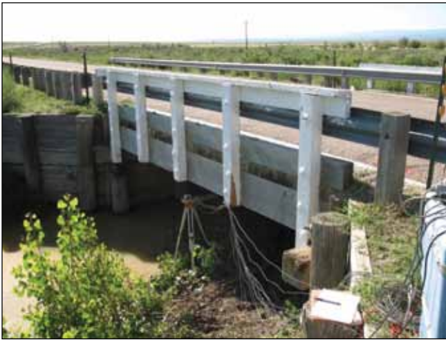
Figure M3. Colorado Bridge parapet support.
