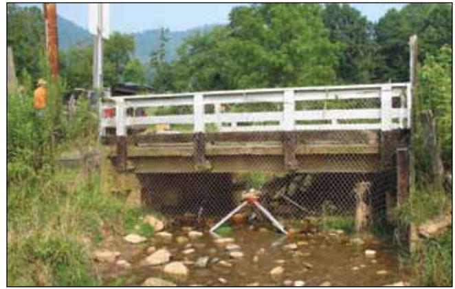
Figure 8. North Carolina bridge used for finite element modeling.
