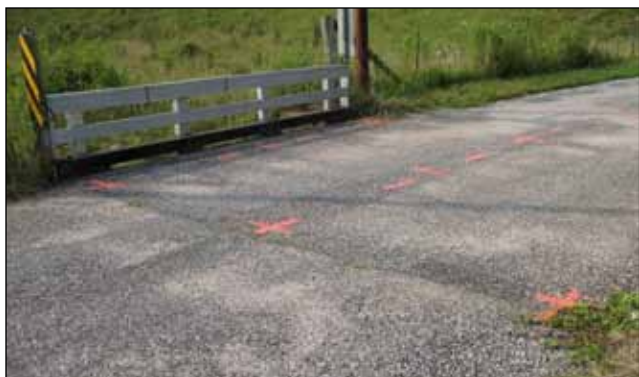
Figure E13. Pavement condition.
