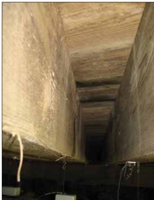
Figure H14. Typical superstructure condition.
