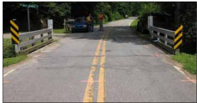
Figure F2. Madison County Bridge.
