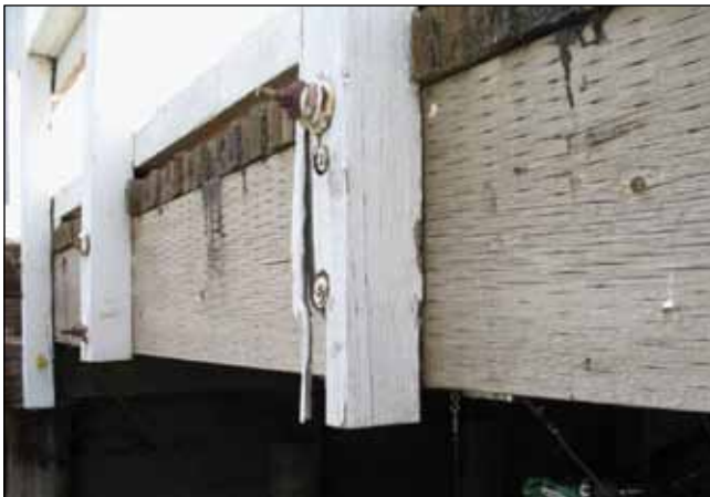
Figure K15. Exterior girder condition.
