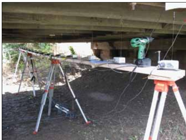
Figure K6. Deflection instrumentation.
