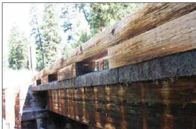
Figure Q3. Trapper Creek Bridge parapet support.
