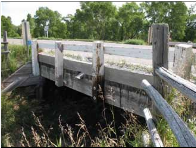
Figure N3. Montana Bridge parapet support.
