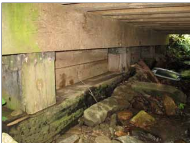
Figure F3. Madison County Bridge substructure.
