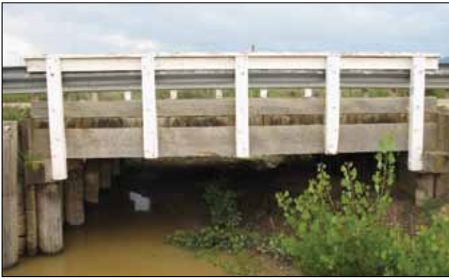
Figure 18. Colorado bridge used for finite element modeling.
