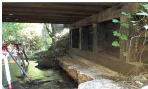
Figure G2. Dix Creek Bridge substructure.
