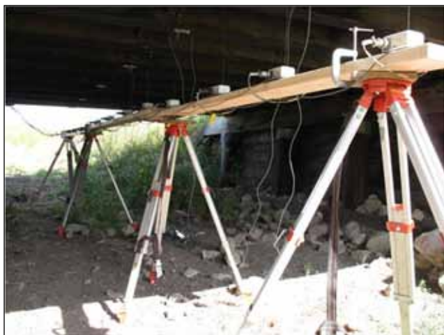
Figure N6. Deflection instrumentation.
