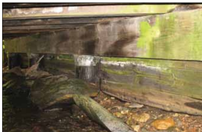
Figure I2. Substructure sill and posts.
