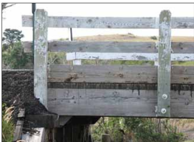
Figure O3. Montana Bridge parapet support.
