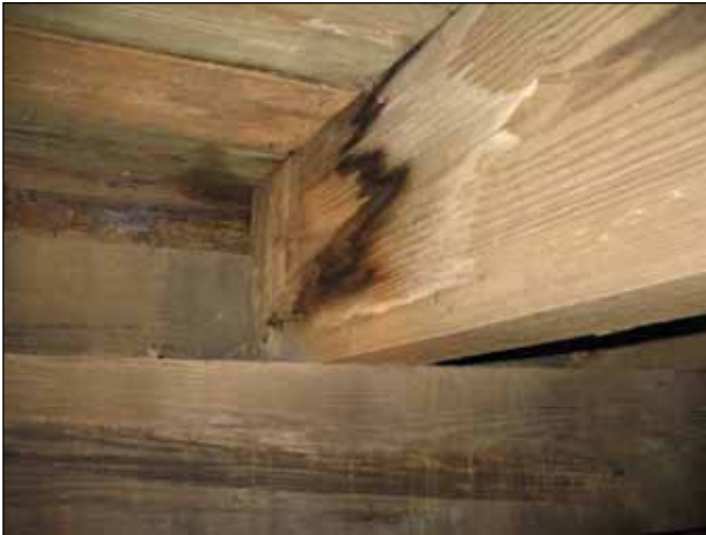
Figure G14. Girder end conditions.
