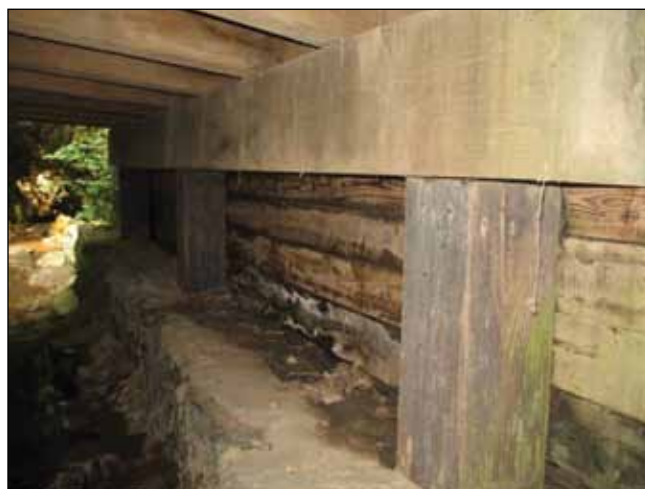
Figure D2. Substructure sill and columns.
