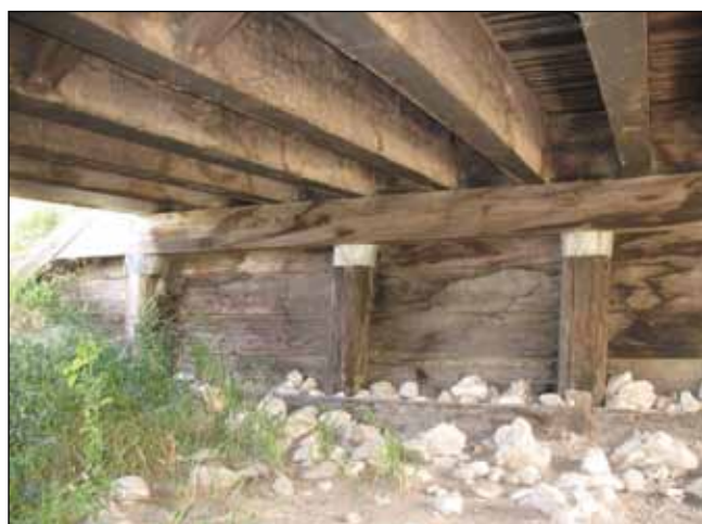
Figure N2. Bridge substructure.
