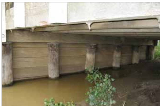
Figure M2. Bridge substructure.
