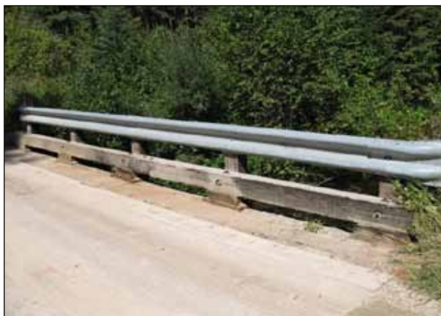
Figure P3. Burnt Fork Bridge parapet support.
