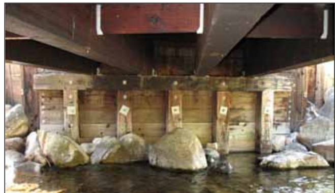
Figure Q2. Bridge substructure.
