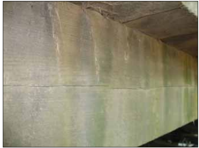
Figure G15. Checking at girder centerline.
