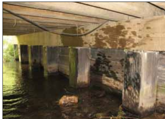
Figure H2. Bald Creek Bridge substructure.
