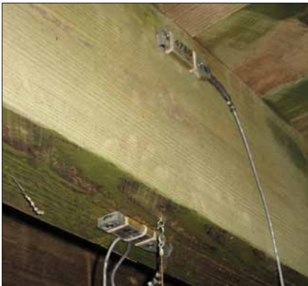
Figure F7. Outside girder strain transducer setup.
