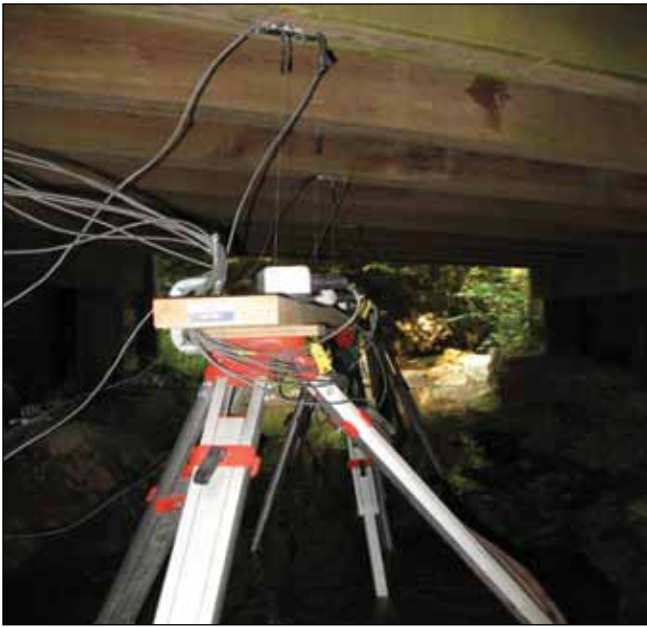
Figure D6. Deflection instrumentation.
