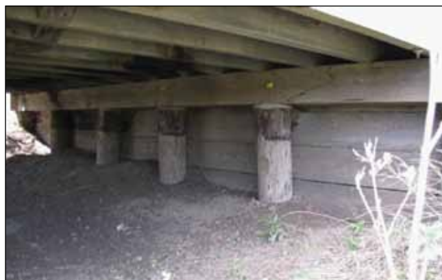
Figure K2. Bridge substructure.
