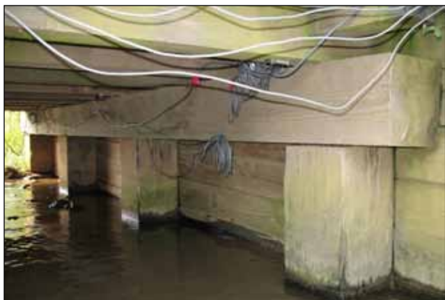
Figure E3. Bridge substructure.
