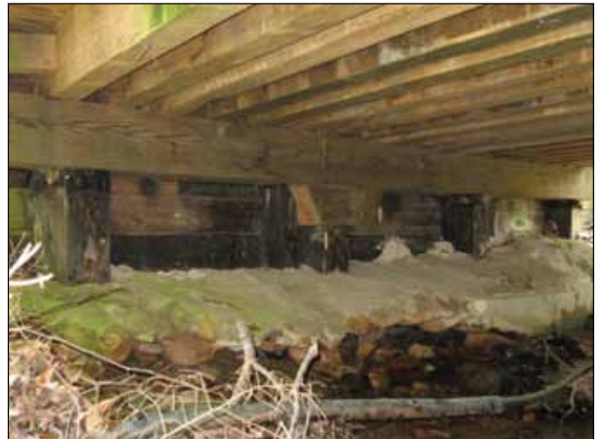
Figure J2. McDowell County Bridge substructure.
