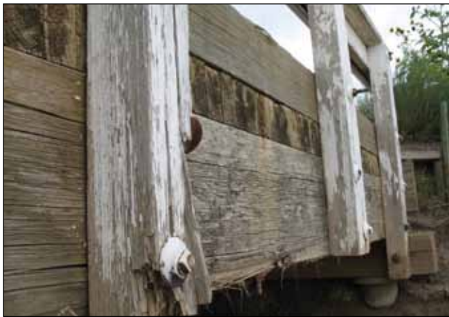
Figure L3. Colorado Bridge parapet support.
