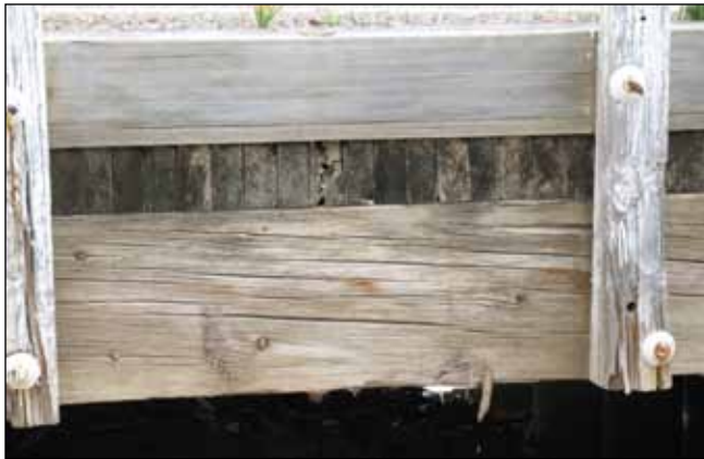
Figure L14. Checking in exterior girders.
