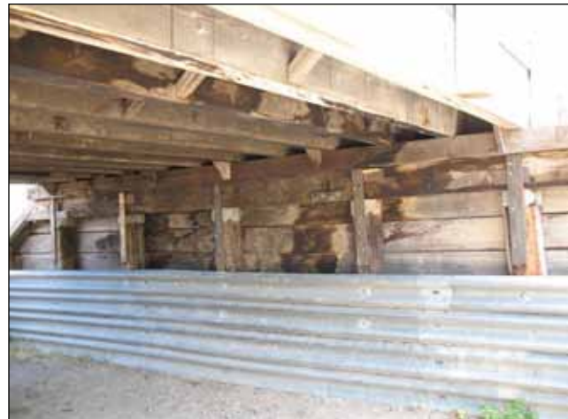
Figure O2. Bridge substructure.
