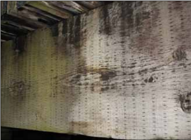
Figure P15. Checking in exterior girders.
