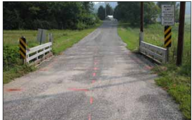
Figure E2. Red Horse Creek Bridge.
