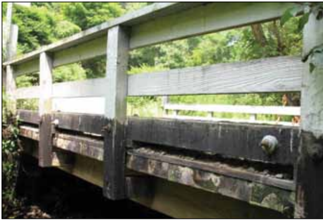
Figure I3. Doebag Creek Bridge parapet.
