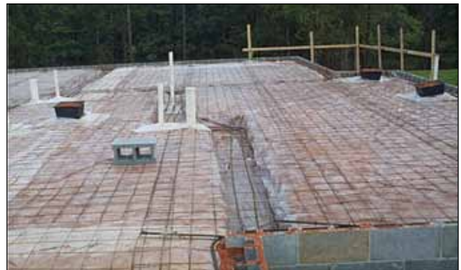
Figure 3—Stem wall foundation with slab prepared for concrete placement, Lot 11.
