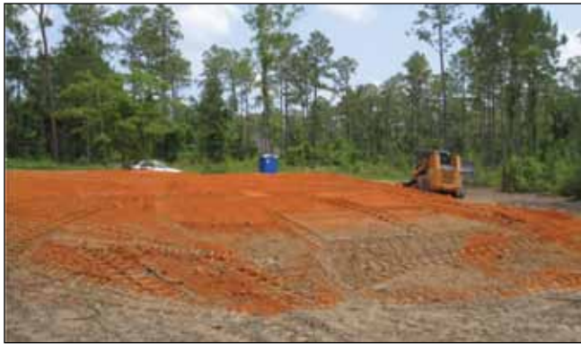
Figure 4—Compacted fill pad, Lot 18 rear.
