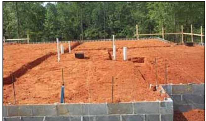
Figure 2—Stem wall foundation with compacted fill, Lot 11.
