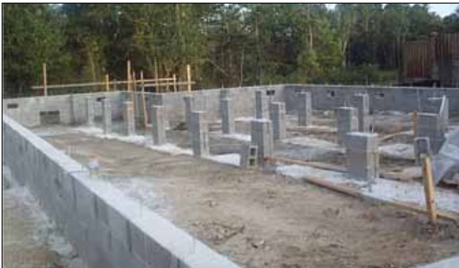
Figure 8—Lot 38 continuous interior footings and piers.
