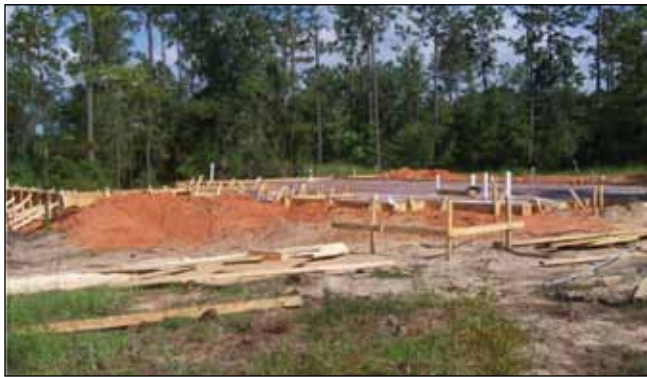
Figure 5—Compacted fill pad prepared for concrete placement, Lot 18 front.
