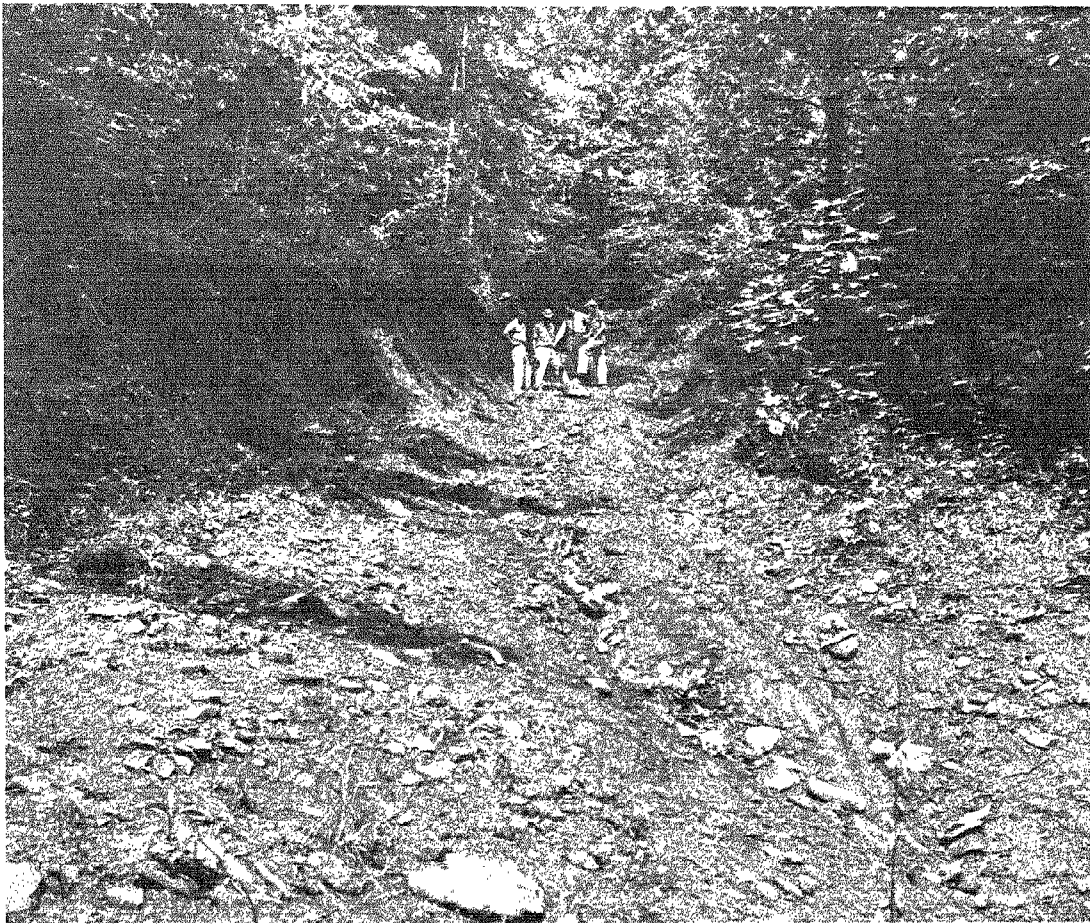
Figure 13.—Several cubic feet of soil were eroded per lineal foot of this carelessly built and managed logging road. Near Franklin, North Carolina, 1952.
