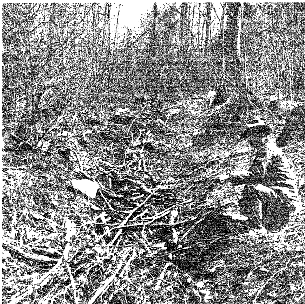
Figure 23. —This entrenched logging road has been packed with logging debris to control further soil erosion. North Carolina, 1950.
