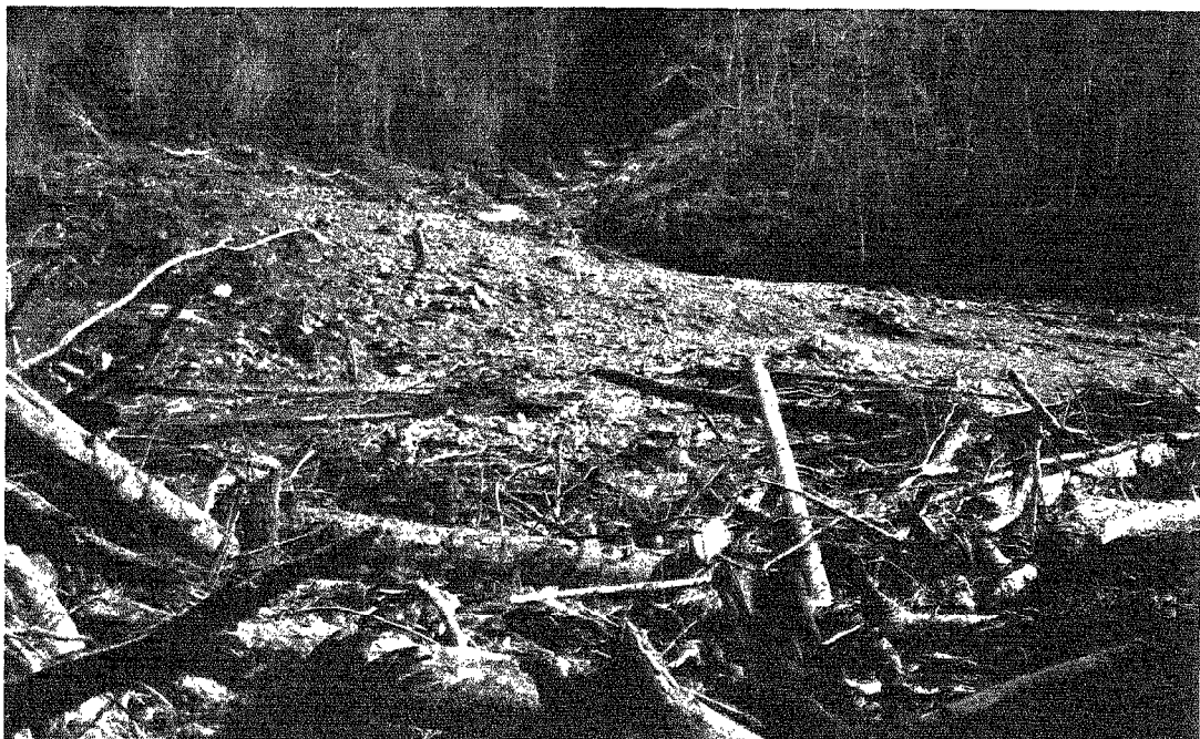
Figure 12.—Carelessly built logging road and landing located too close to a stream. Here, eroded soil quickly becomes stream sediment. Location and date unknown.
