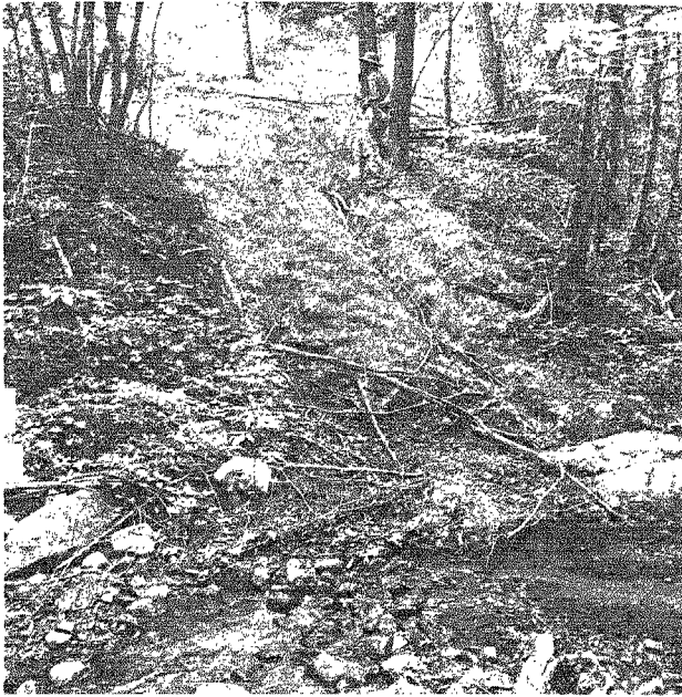
Figure 24.—Erosion control is especially important when soil washed from poorly located roads can be carried directly into streams. Virginia, 1956.
