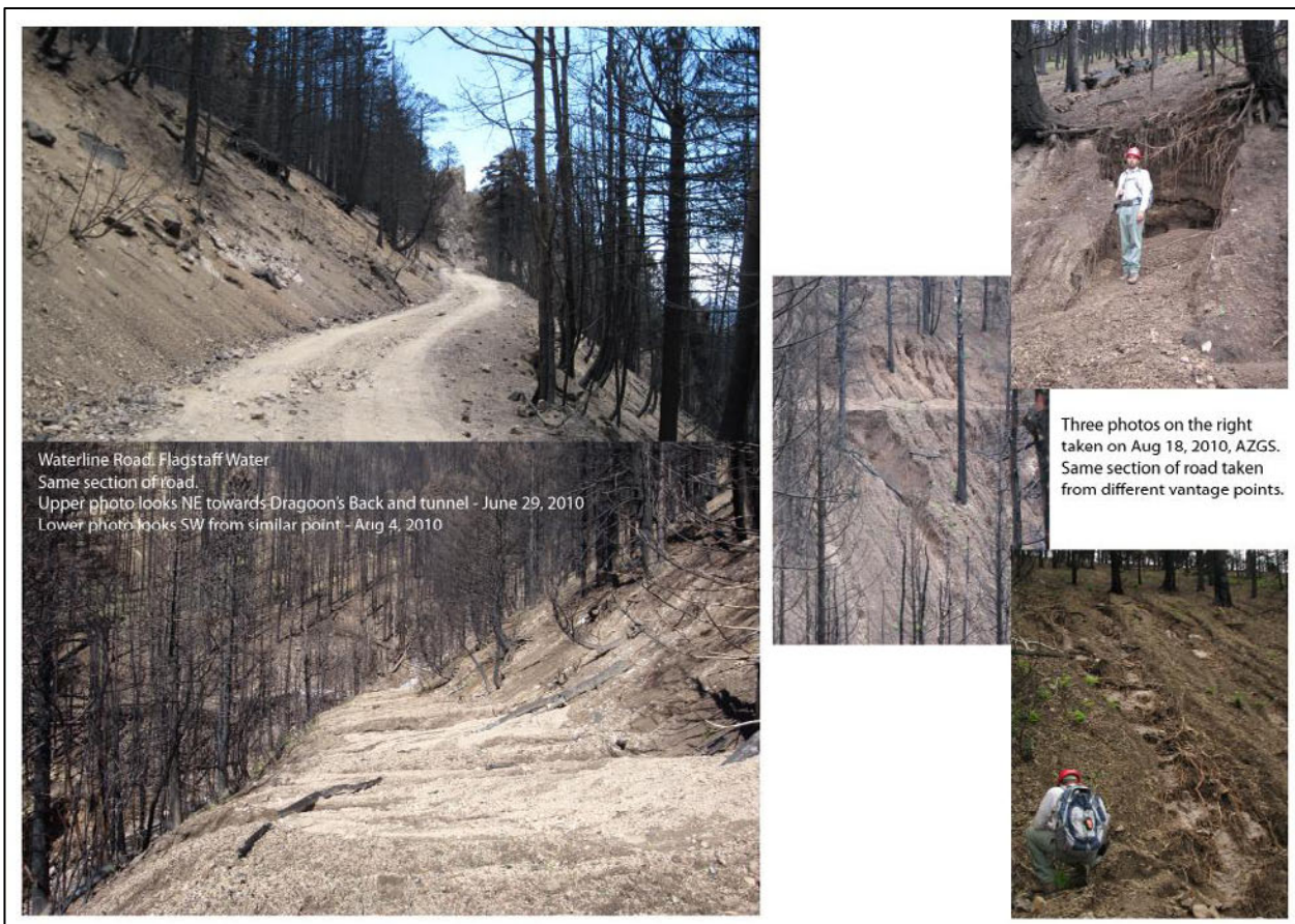
Figure 12. Examples of hillslope erosion along the Waterline Road immediately after the fire (upper left) and after rainfall.
