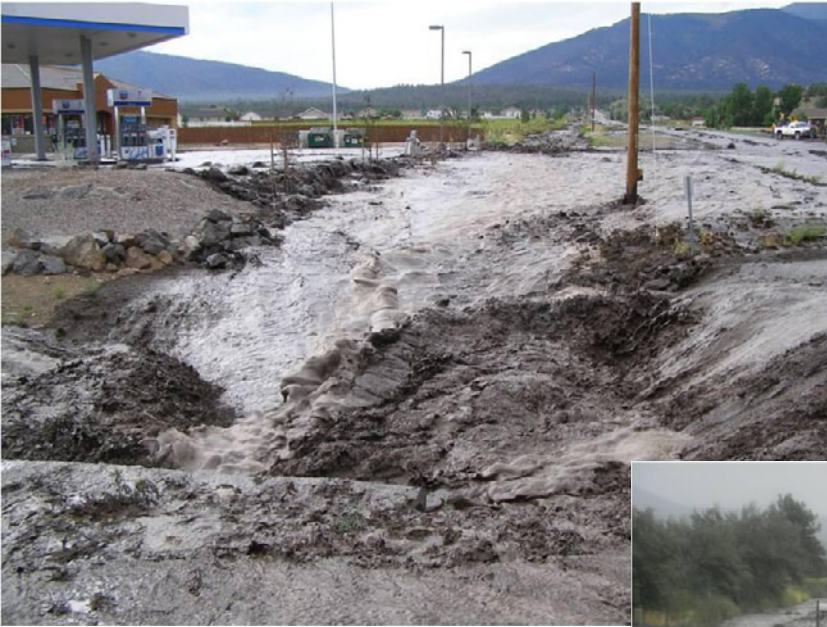
Figure 17 (upper left). Flow from Campbell Avenue and ditch at the Chevron Station, Timberline, during first major post-fire flow event, 20 July 2010 (prior to infrastructure upgrades). Photo: D. Neary US FS RMRS.
