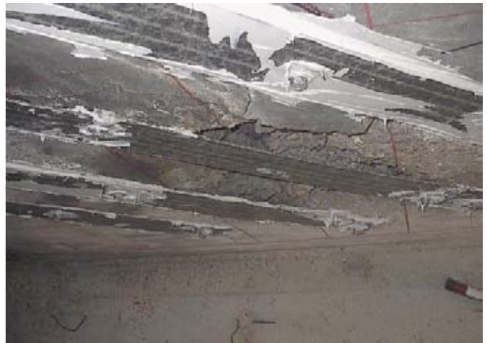
Severe deterioration prevented the application of a bonded strengthening system to this bridge in Pulaski County, Missouri, but MF-FRP applied SAFSTRIP® was able to repair the bridge.
