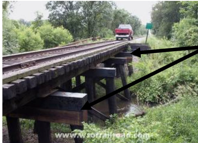
Figure 7: A completed rehabilitation project of bridge F-76 on the WSOR line in the Monroe Subdivision. Note some of the bents have been double capped – the first bent in the foreground and the 4 th bent (Wisconsin & Southern 2008).
