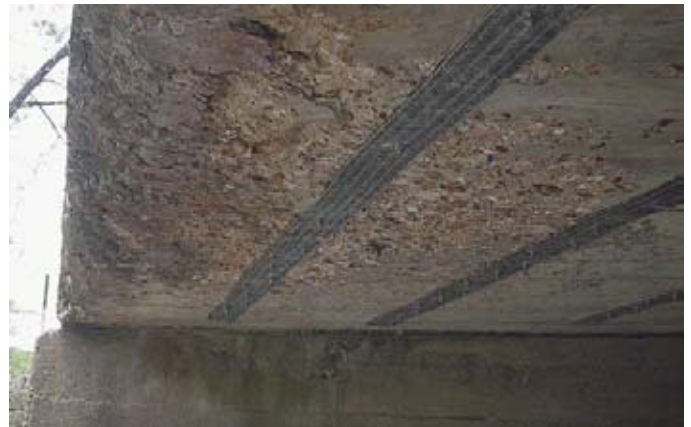
As a result of a SAFSTRIP® retrofit, the existing 12-ton load posting for this bridge in Phelps County, Missouri, was removed.
