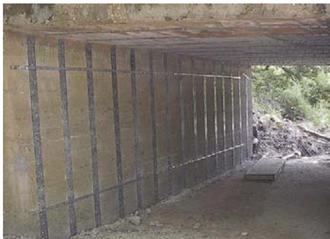
The abutment and deck of this bridge in Phelps County, Missouri, was strengthened using SAFSTRIP®.
