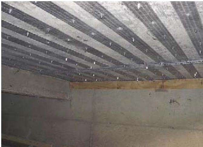
This bridge, located in St. James, Missouri, was load posted at the time of strengthening. After mechanically attaching SAFSTRIP® with concrete wedge bolts and anchors, the bridge load limit was raised to 20 tons.
