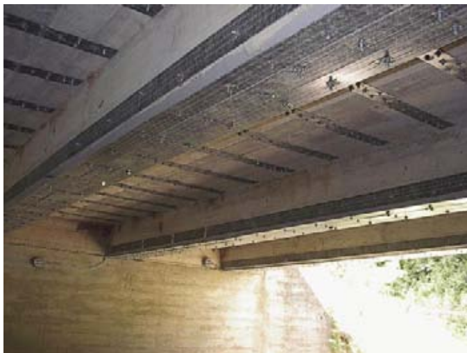
The posted load for this bridge that spans the Meramec River in Missouri was increased from 10 tons to 18 tons by installing SAFSTRIP® using the MF-FRP system.
