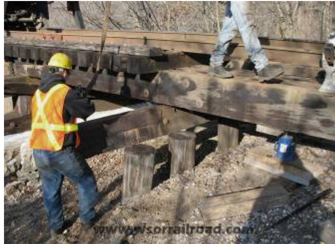
Figure 6: Rehabilitation of a timber bent for a bridge on the WSOR line in the Reedsburg subdivision. The deck was jacked up, and any deterioration in the piles was removed by sawing their tops off. A new pile cap is shown being placed over the piles. In the case of bridges which are double capped, a second pile cap would be stacked with the first (Wisconsin & Southern 2008).
