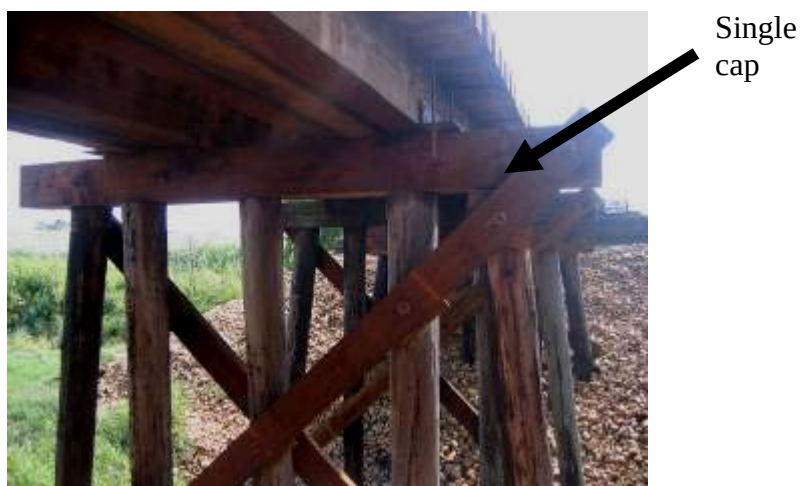
Figure 3: Bridge F-134 on WSOR operated line showing a single pile cap.
