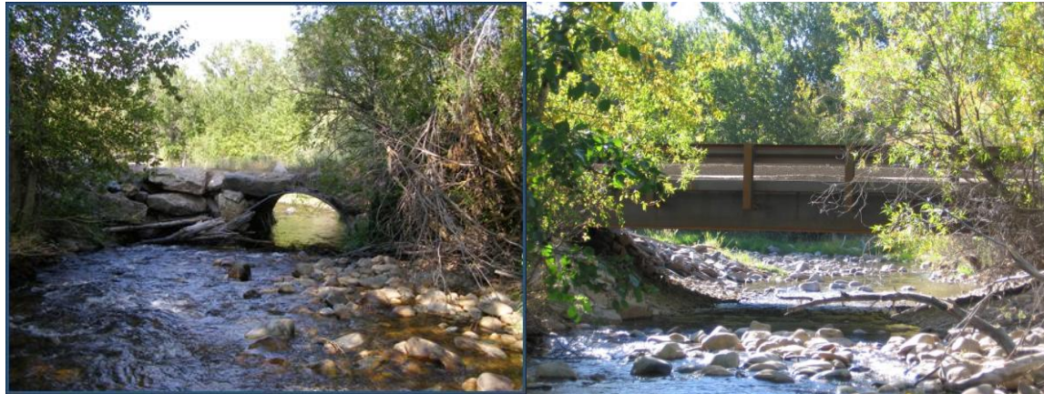
Figure 2 - Parmenter Lane road crossing before and after culvert to bridge replacement.
