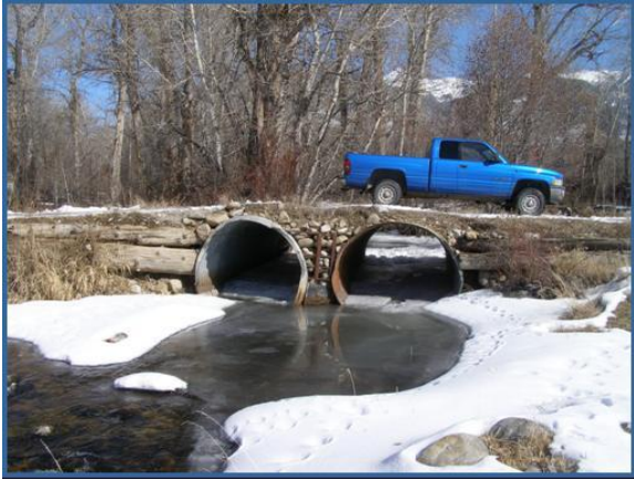
Figure 3 - Archie Lane road crossing before culvert to bridge replacement. Bridge here similar to Parmenter Lane.
